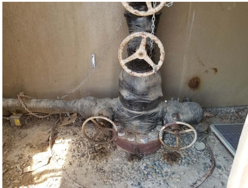
Photo 2. No bradenhead access apparent.
