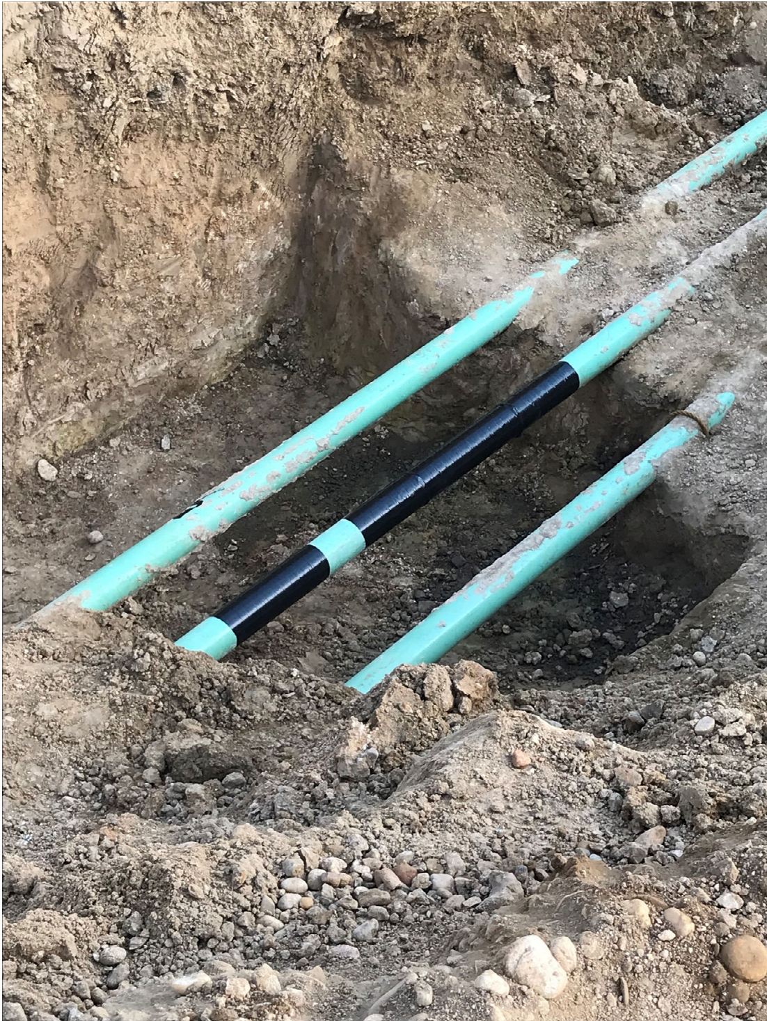
Photo Taken 8/31/2021 – Photo taken following replacement of compromised section of flowline.
