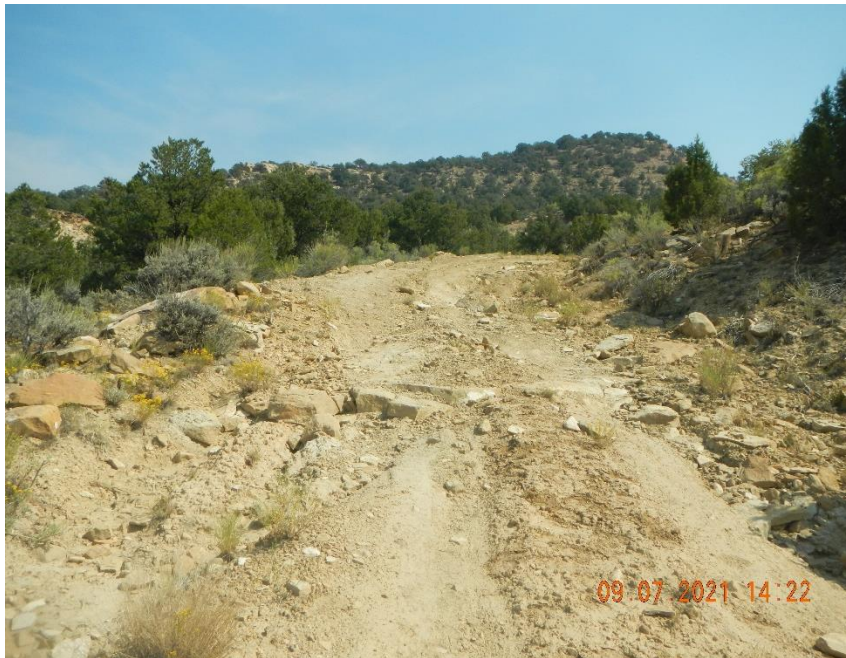
Storm water washing access road and ditches.
