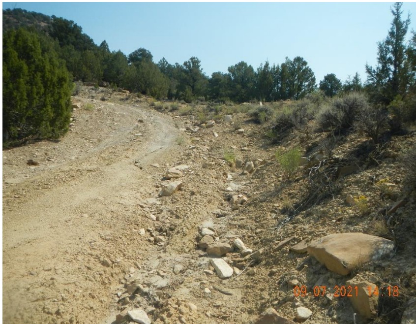
Storm water washing access road and ditches.
