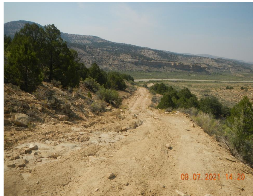
Storm water washing access road and ditches.
