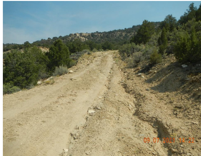
Storm water washing access road and ditches.
