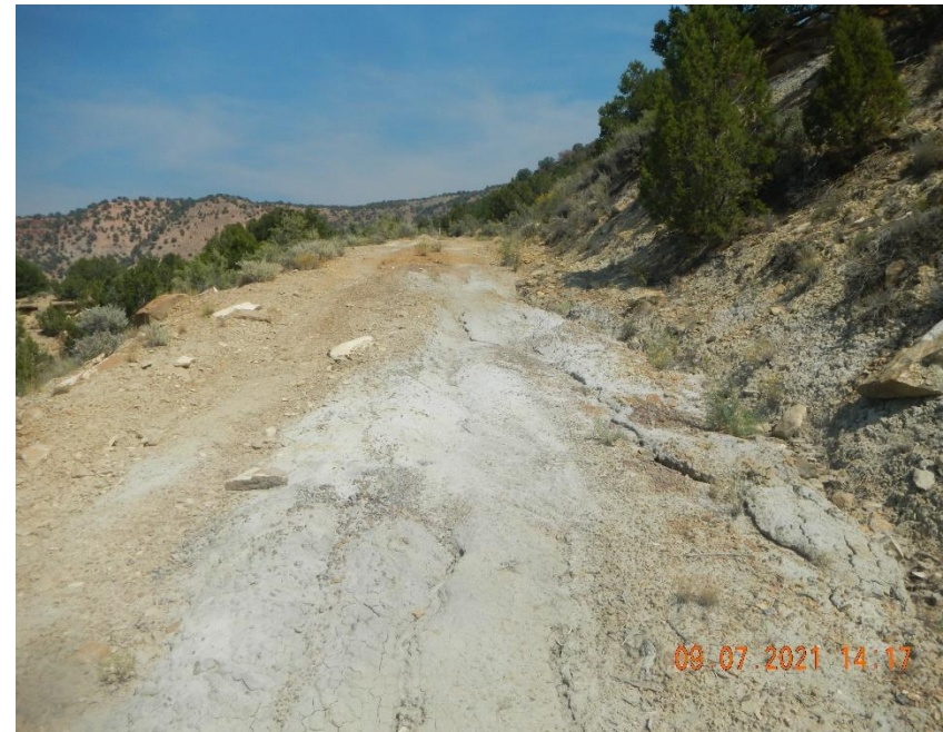
Storm water washing access road and ditches.
