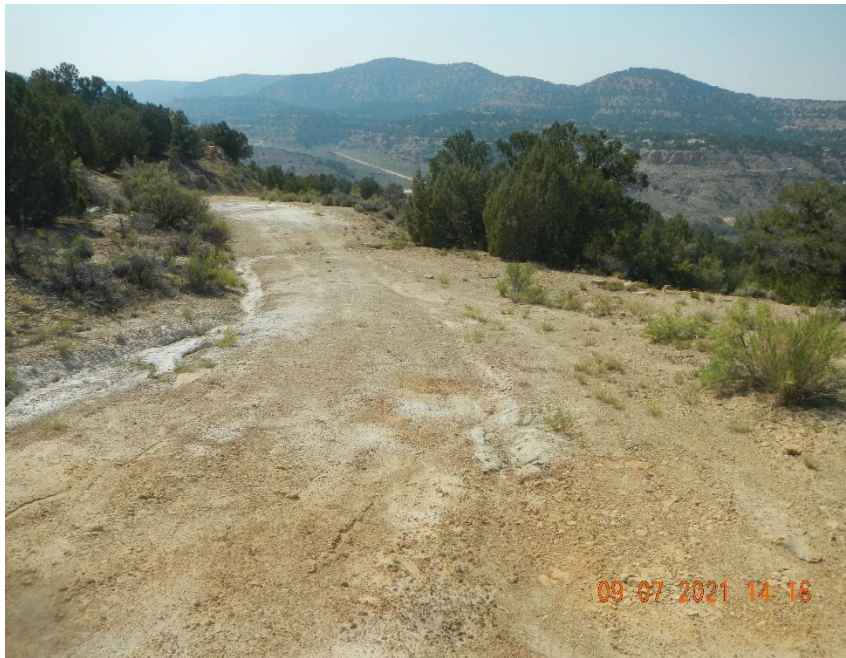
Storm water washing access road and ditches.
