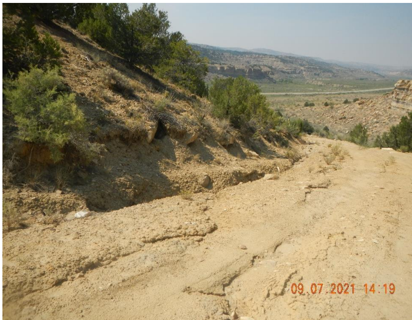
Storm water washing access road and ditches.
