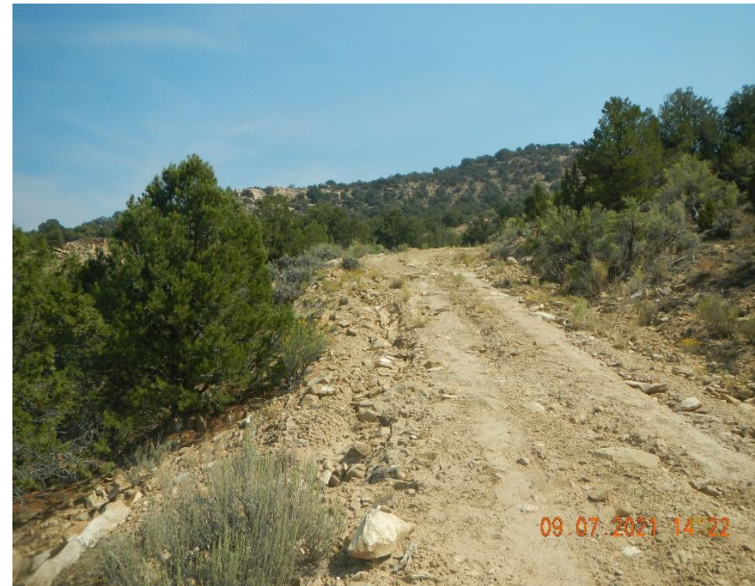
Storm water washing access road and ditches.
