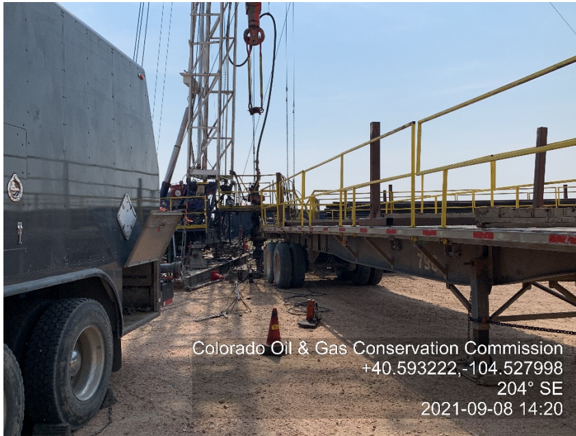
Photo #1 Cummins AB 10-1IJ (05-123-30293) Wellsite Plugged & Abandoned | PA Plugging Operations: Cementing | Initial Plugs
