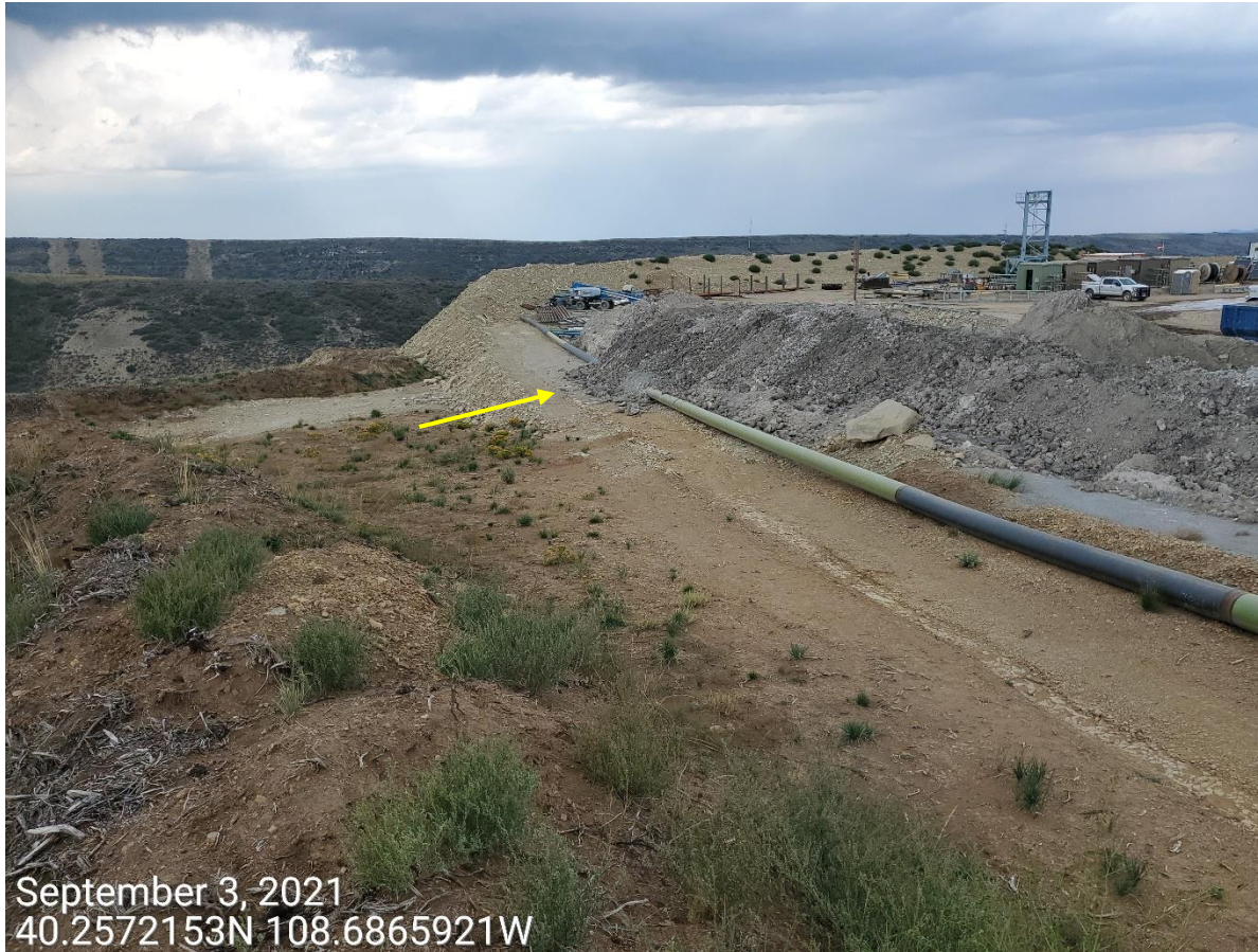
Photo 1: Photo taken from the south end of the Location, facing west. Photo shows control measures to contain drill cuttings is missing, or inadequate. Areas observed on the left of the photo include the perimeter stormwater controls (retention pond) for the Location
