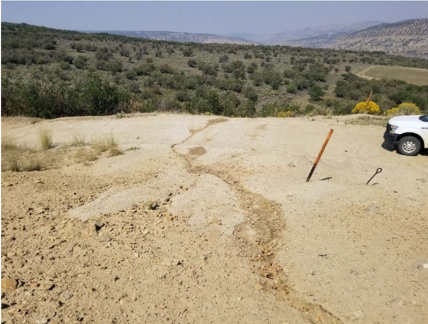
Photo 7. Erosion compromising berm and moving sediment to location perimeter.
