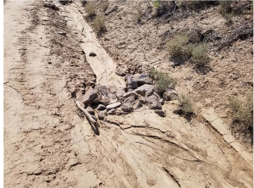
Photo 10. BMPs full of sediment in access road ditch.
