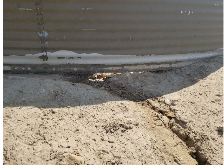
Photo 6. Berm compromised by erosion.
