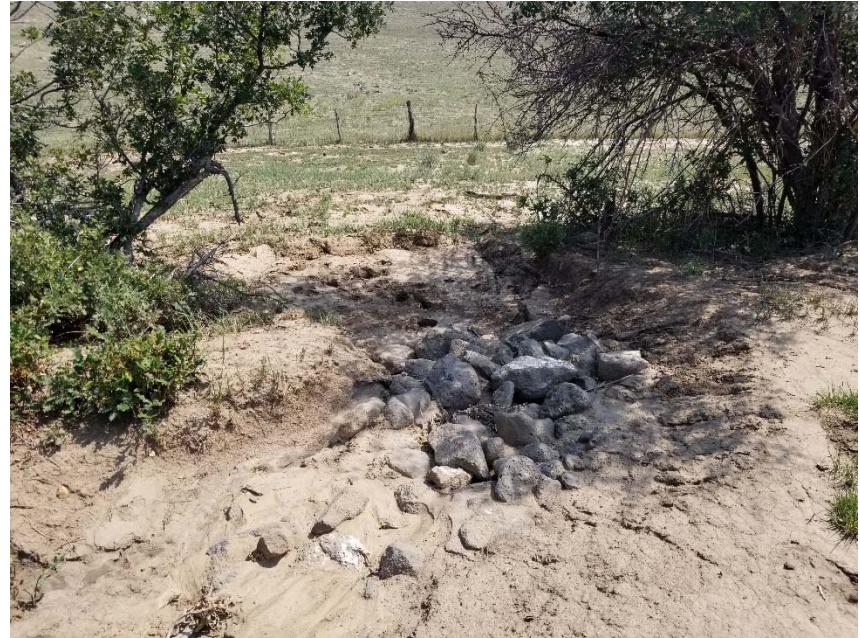
Photo 12. BMPs full of sediment, sediment moving off access road.
