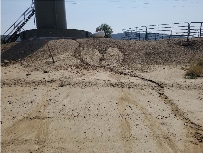
Photo 5. Erosion compromising berm and moving sediment to location perimeter.
