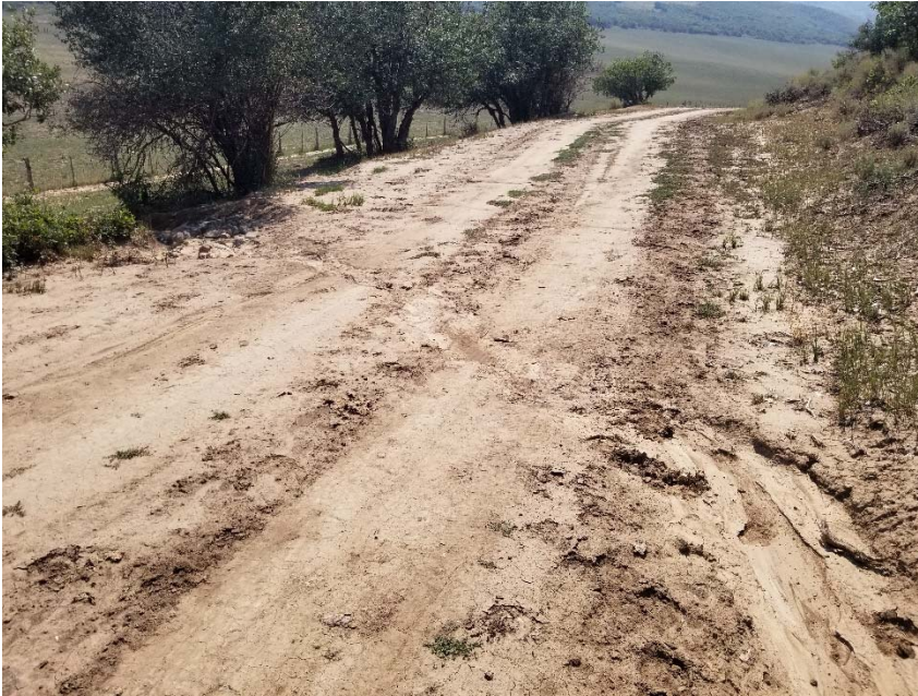
Photo 11. Sediment moving out of ditch, across access road, and off of access road.
