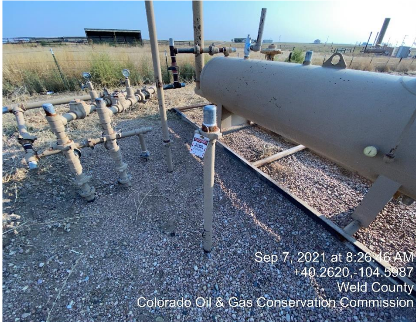
Photo #3 Tagged riser but isn't marked
