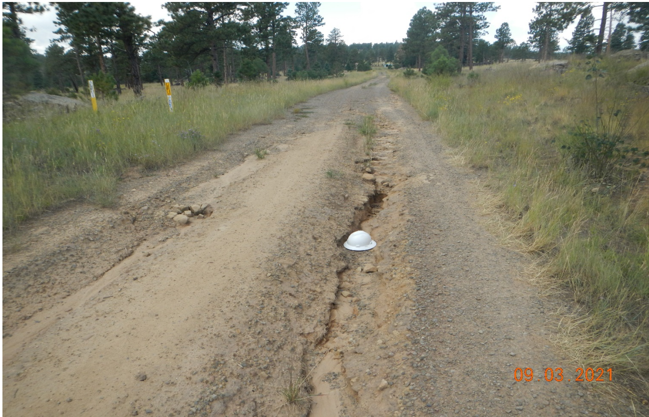
Photo 2. Facing southwest along the access road. There area areas of erosion along the road. Hard hat was placed in erosion channel for scale.
