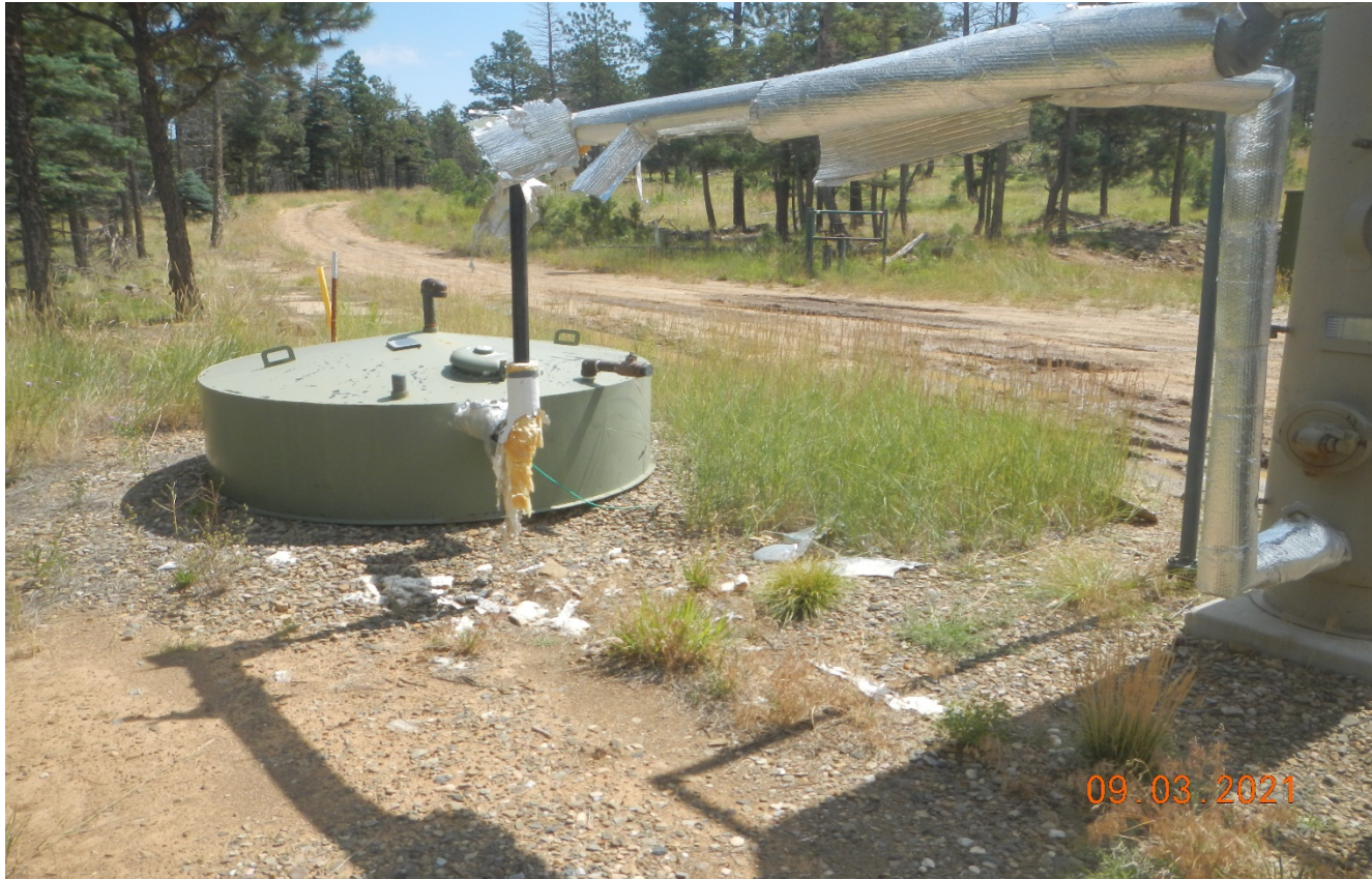
Photo 9. The insulation around the piping is degraded. The insulation debris needs to be cleaned up and removed.
