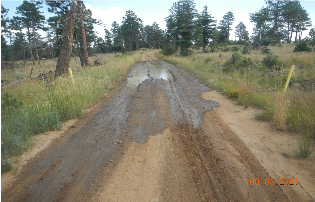
Photo 4. Likewise to previous photo. There is a low spot in the road where stormwater accumulates and vehicles are widening the road to avoid this area. This area needs to be repaired to allow proper drainage.
