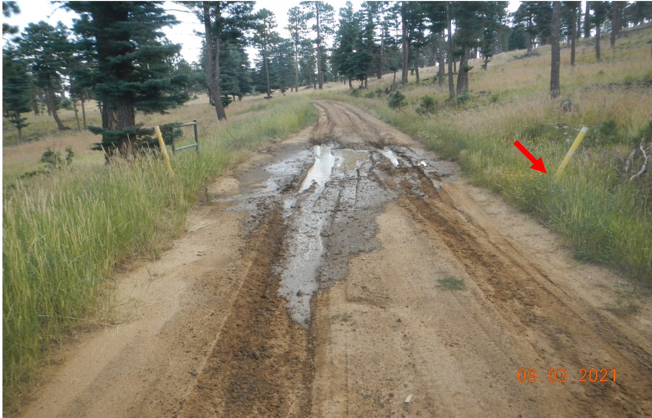
Photo 3. Facing southeast along the access road. There is a low spot in the road where stormwater accumulates. This area needs to be repaired to allow proper drainage. Red arrow points to culverts that are not maintained to allow proper drainage.
