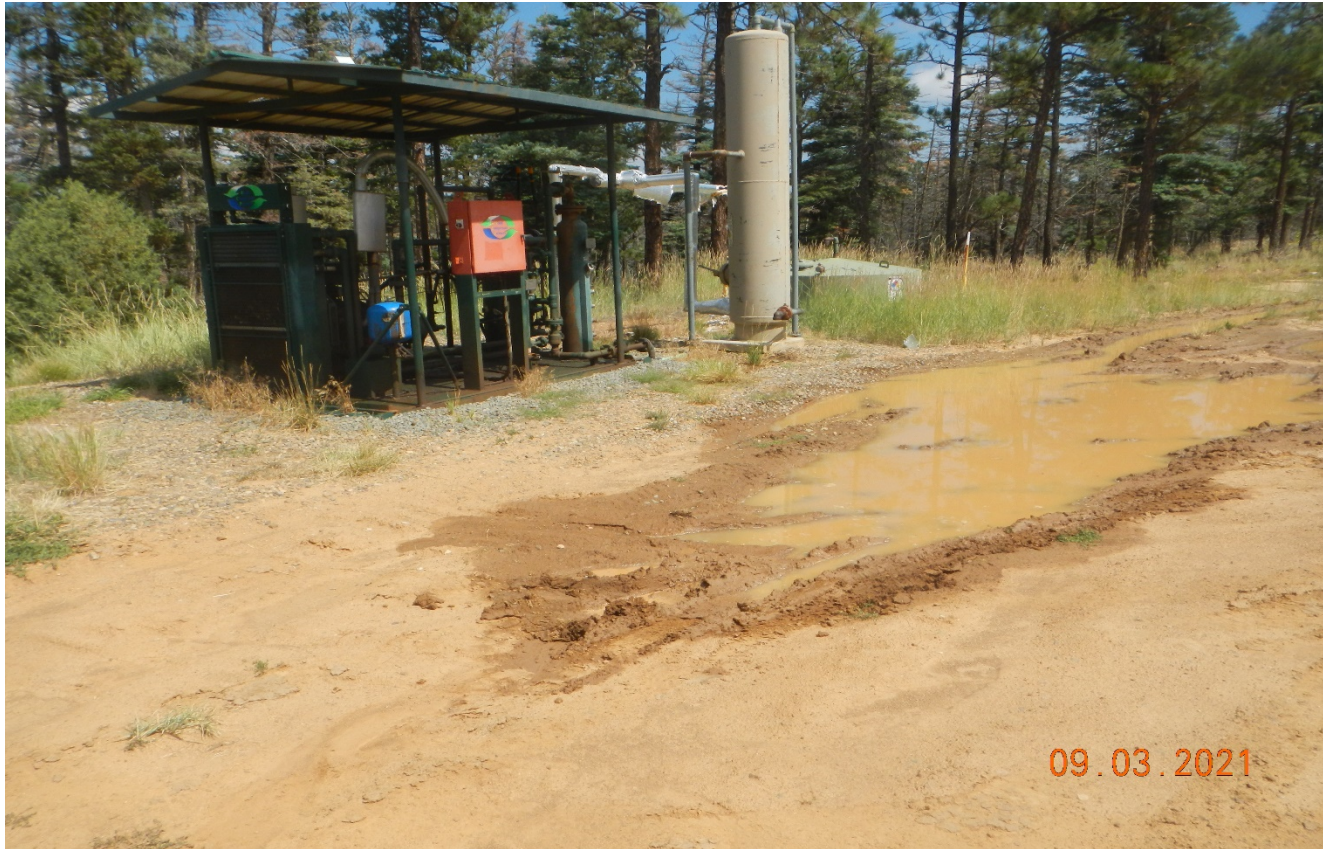
Photo 8. Facing toward the location. Areas of rutting at the location need to be repaired and stabilized. Production areas are not stabilized.
