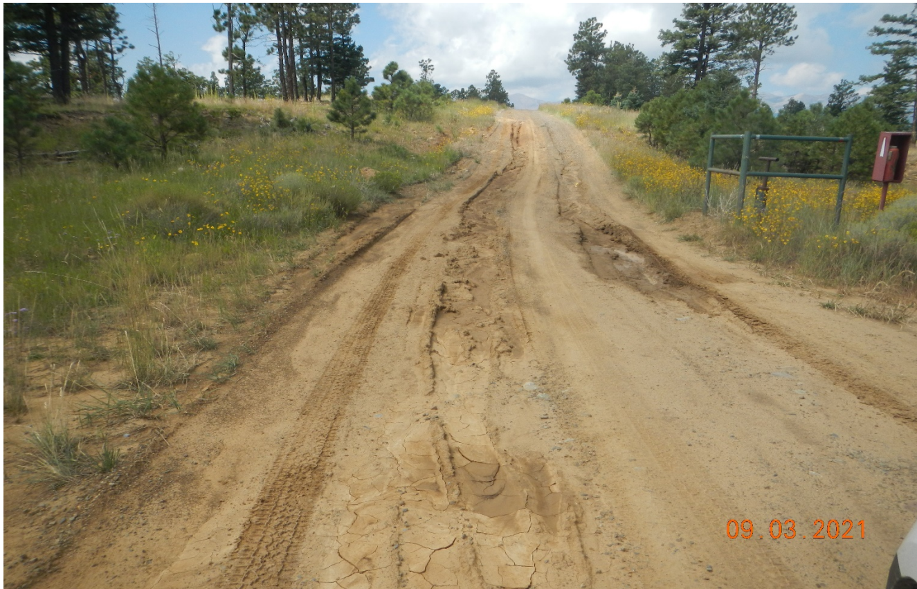
Photo 1. There is vehicle rutting along the road traveling to the location. The road needs to be maintained. Previous corrective action has not been completed.
