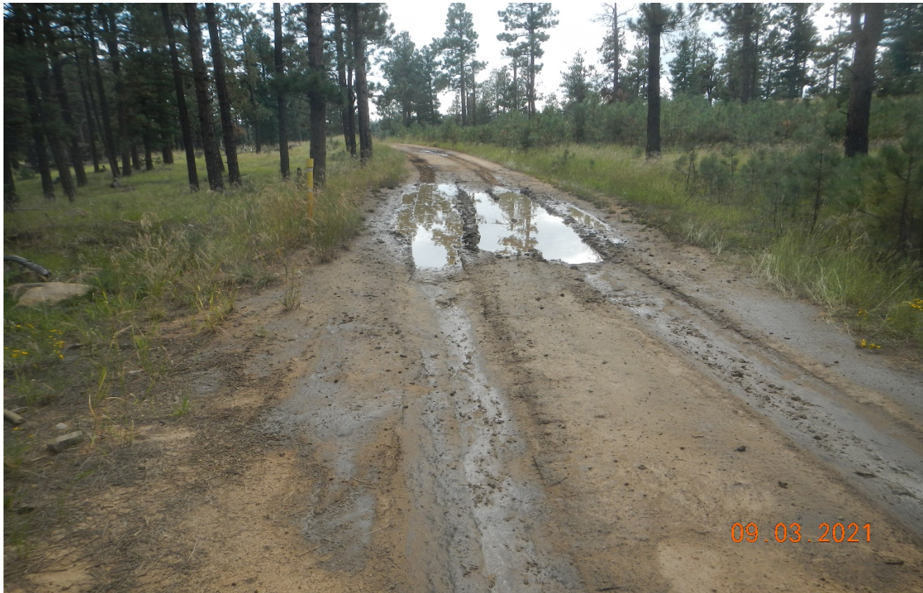
Photo 6. There is vehicle rutting along the road traveling to the location. The road needs to be maintained.
