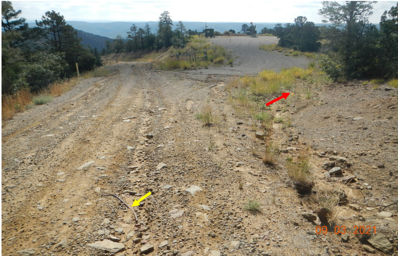
Photo 2. Stormwater is directed down the road causing erosion shown in previous photos. Stormwater should be diverted off the road shown at red arrow, The yellow arrow points to a piece of rebar stuck in the road which could puncture a tire.
