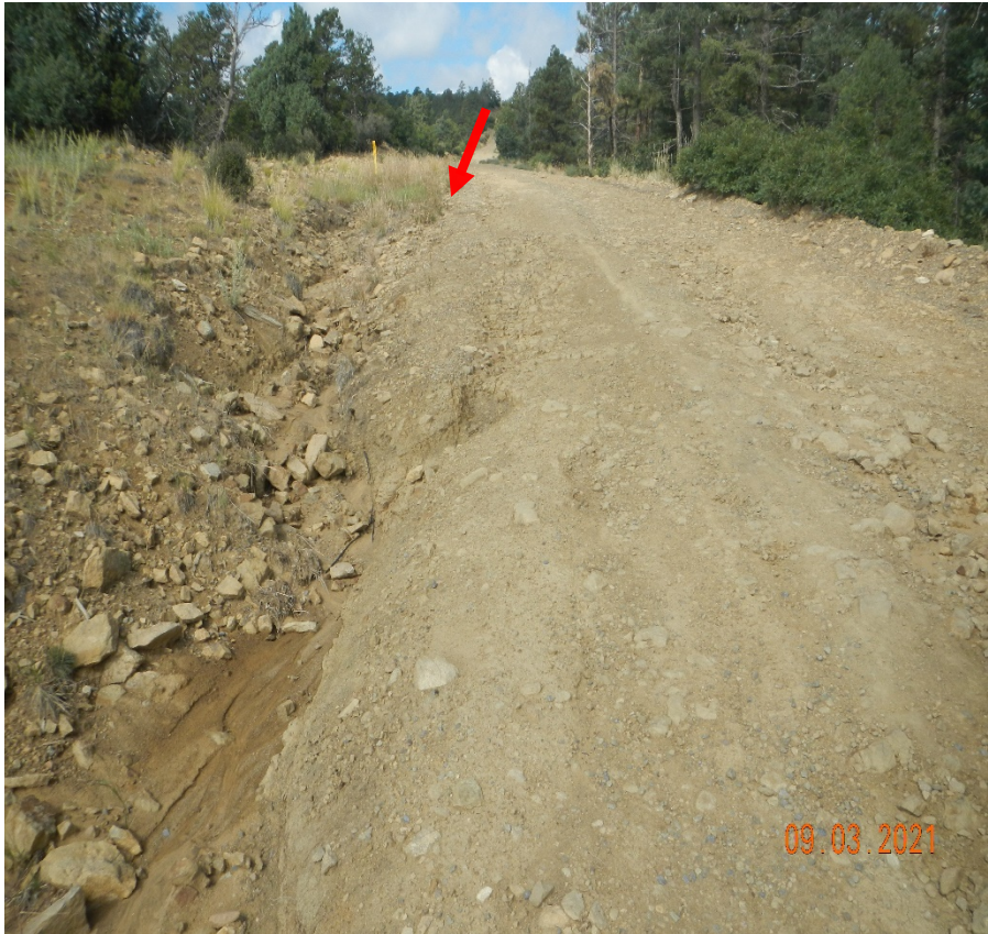
Photo 1. Facing west along the access road. There is insufficient BMP's along the road causing stormwater to flow down a long portion of the road which is causing erosion. Previous corrective action was not performed.
