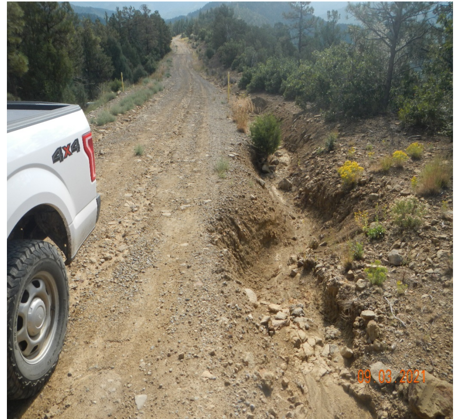
Photo 1. Facing west along the access road. There is insufficient BMP's along the road causing stormwater to flow down a long portion of the road which is causing erosion. Previous corrective action was not performed.
