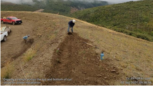
Installing Trenches to Anchor Upper and Lower Ends of Erosion Control Blanket Installations
