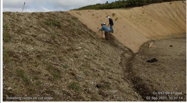
Installing Erosion Control Blanket on the Cascade Creek 697-09-61 Pad
