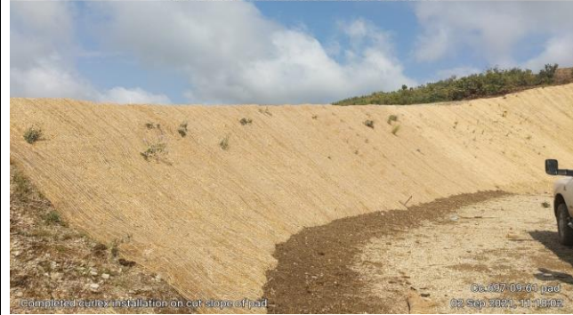
Erosion Control Blankets Installed on the CC 697-09-61
