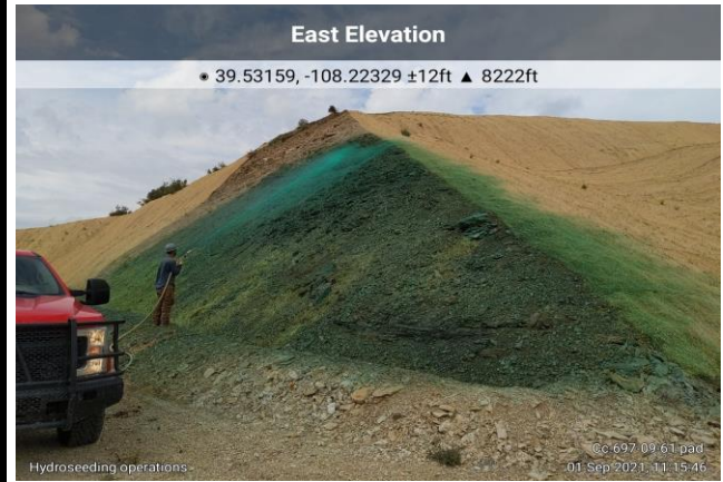
Applying Liquid Nutrients to Steep Cut Slope on the CC 697-09-61 Pad
