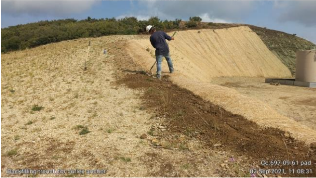
Backfilling Trench on CC 697-09-61 Pad
