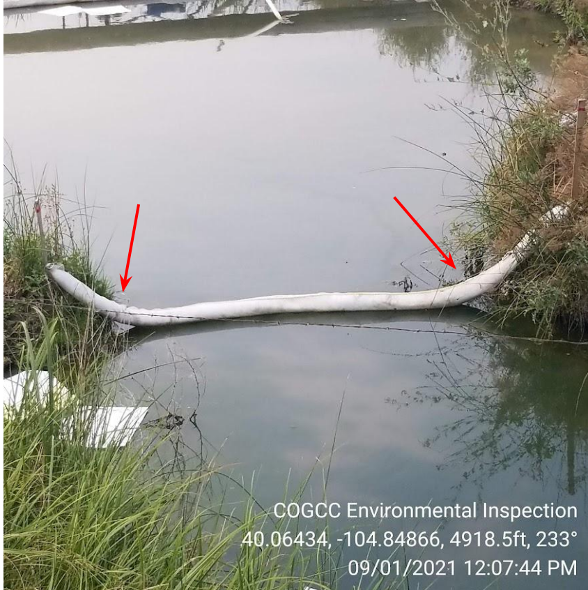
Photo 17 – Upstream of culvert; booms deployed with visible gaps under allowing product to bypass controls.
