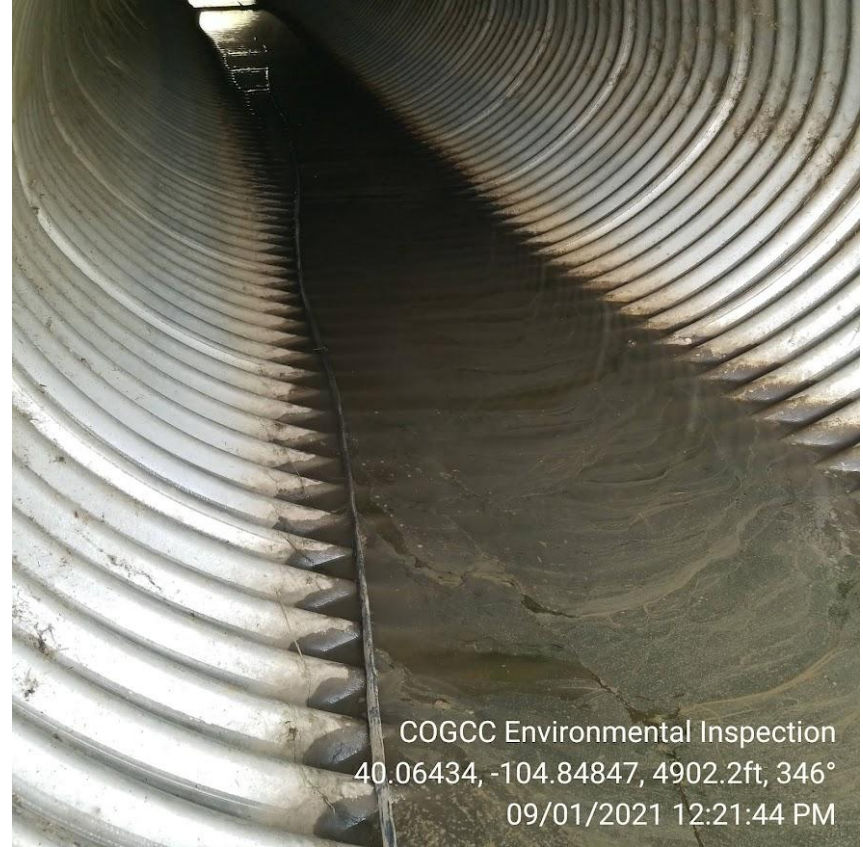
Photo 20 – Culvert under County Road 23. Hydrocarbon impacts visible.
