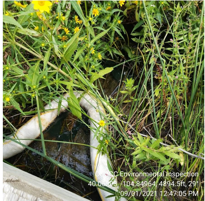
Photo 4 – Boom deployed in wetland, gross free product visible.
