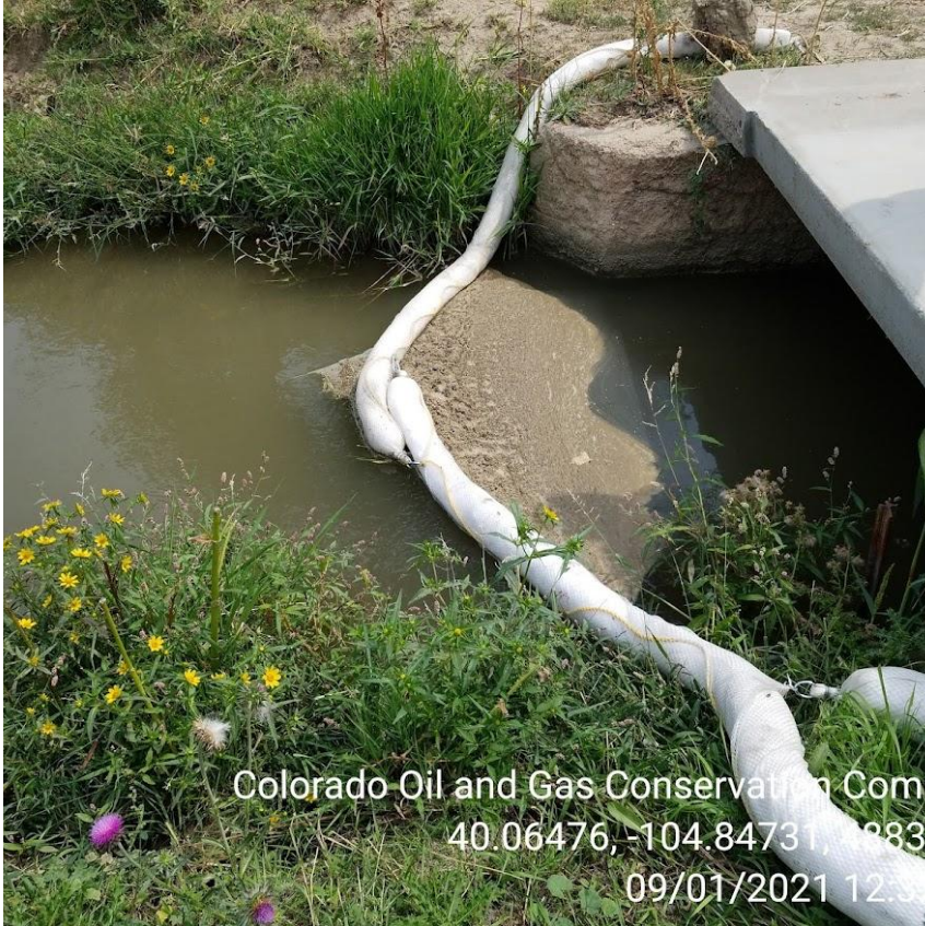
Photo 27 – Boom on irrigation canal.
