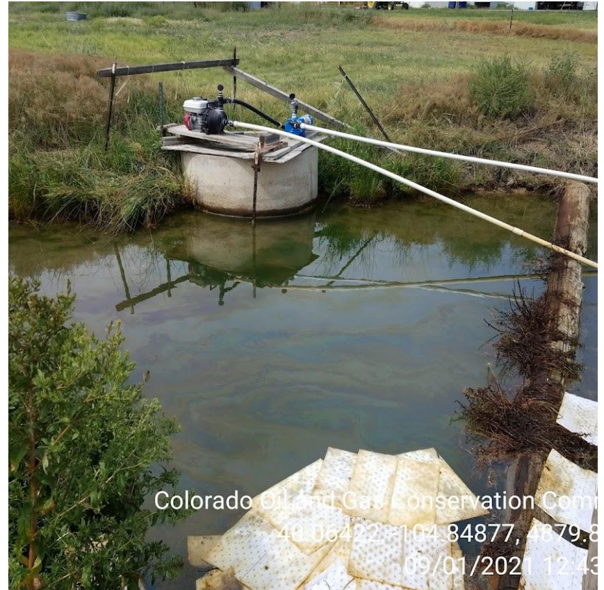
Photo 14 –Cistern pumps adjacent to booms.
