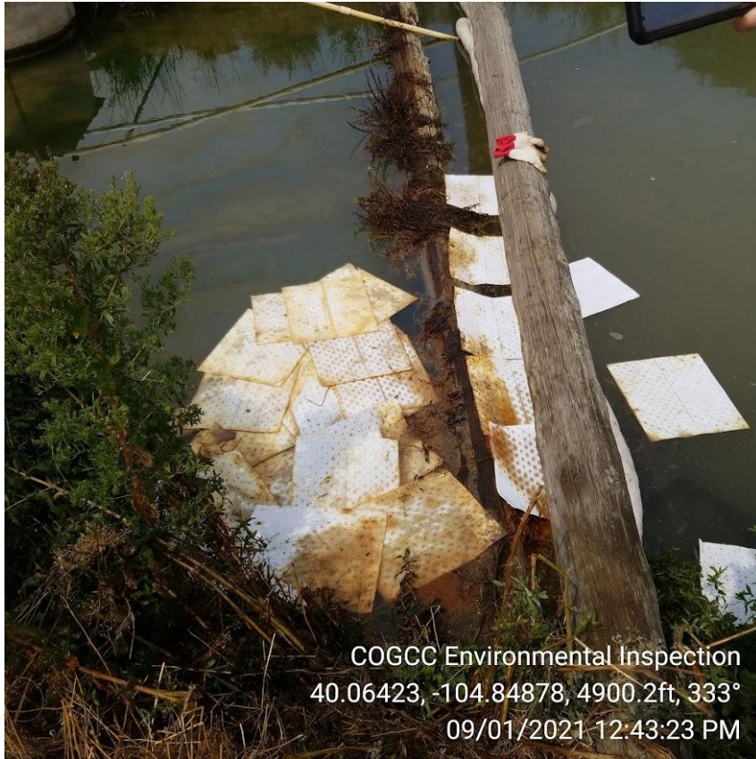
Photo 13- Gross free product visible in wetlands, absorbent pads and boom placed by operator.
