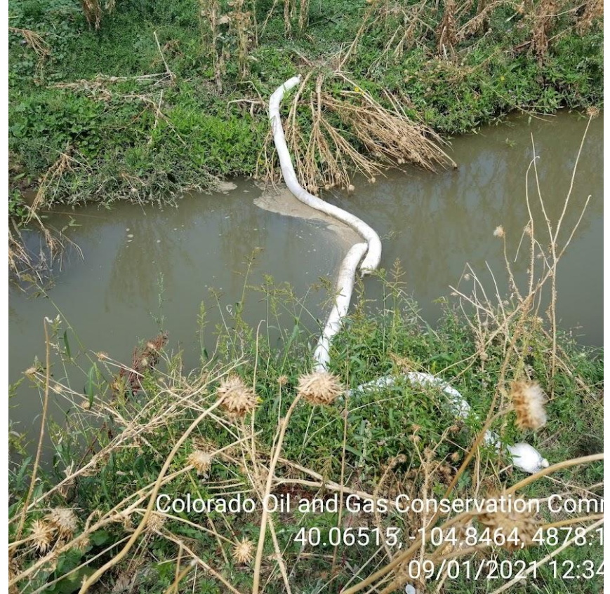
Photo 28 – Final boom on irrigation canal.
