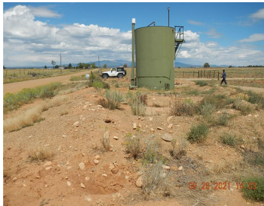
Weeds and animal burrows within secondary containment berm.
