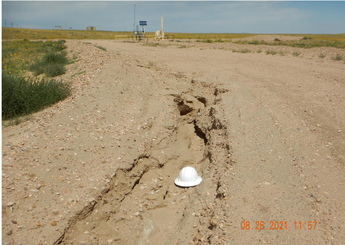
Photo 5. Photo taken from the southern access road, facing North. Photo illustrates gully erosion in need of repair.
