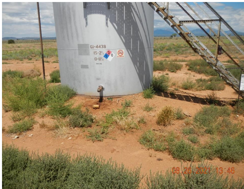
Stained soil beneath AST load out valve. Weeds present within secondary containment berm. Contents are not labeled.
