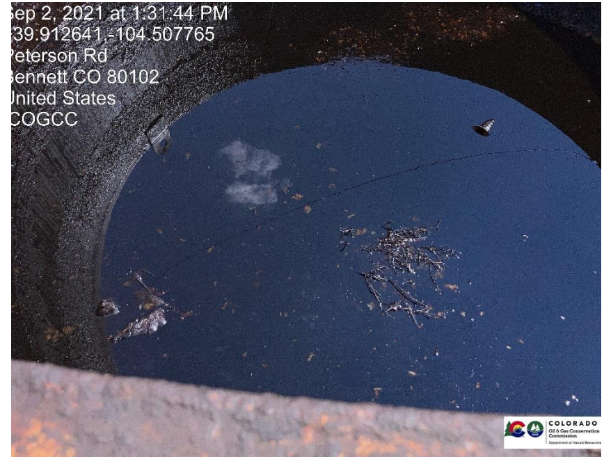
Pic 8 what appears to be dead animals in open top tank, oil present in open top tank, no netting, or content, placard, volume signs.
