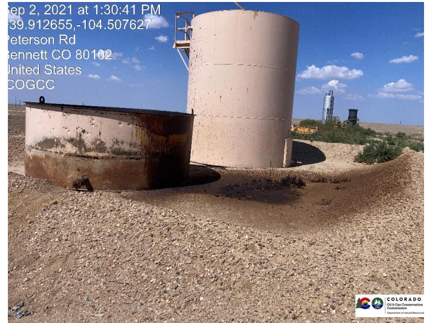
Pic 6 spill from open top tank approx. 20'X14'
