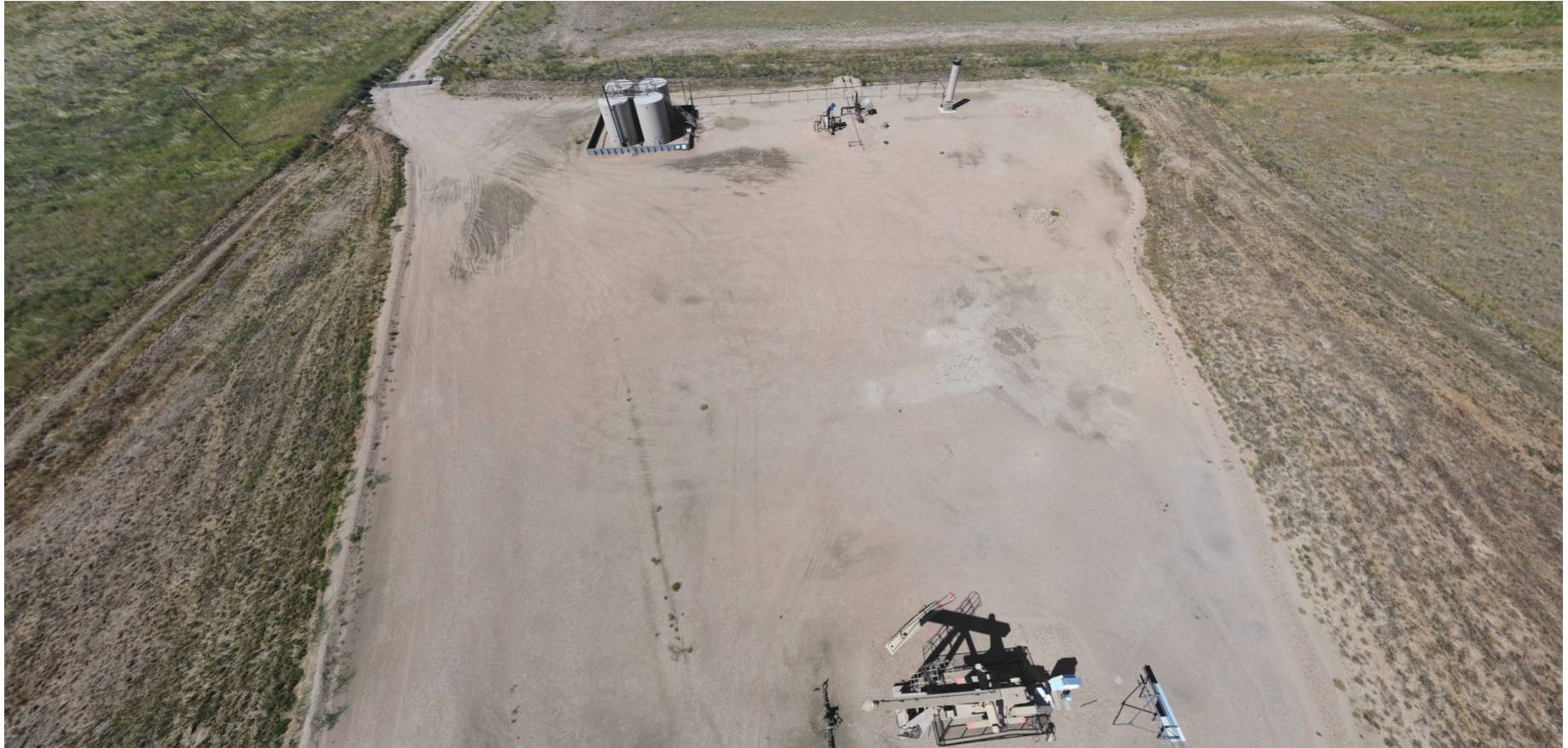
Photo 3. Drone aerial imagery illustrates the well location and the western location. See comments under Photo 1.
