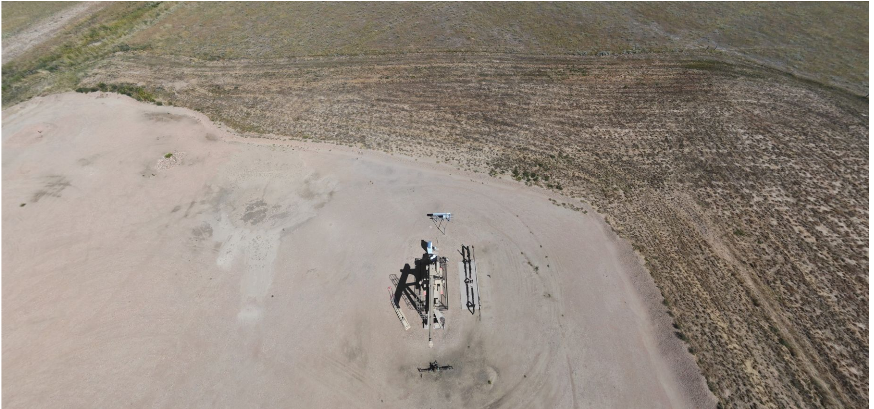
Photo 4. Drone aerial imagery illustrates the multi-well location and the northern location. See comments under Photo 1.
