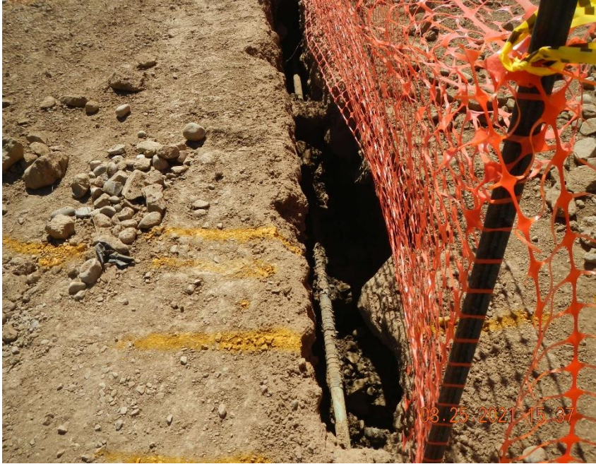
Flow line in open trench.
