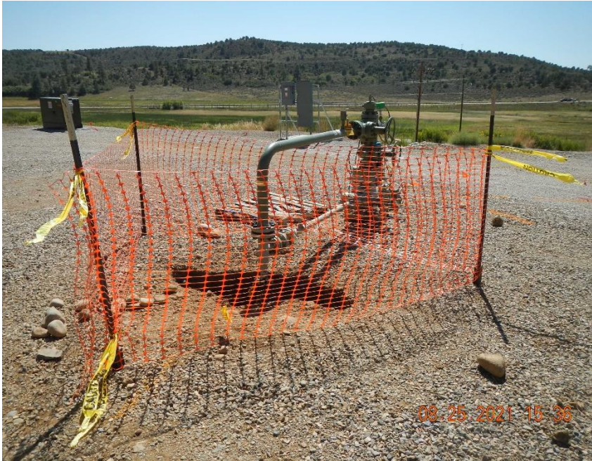
Excavation around flow line at well head.
