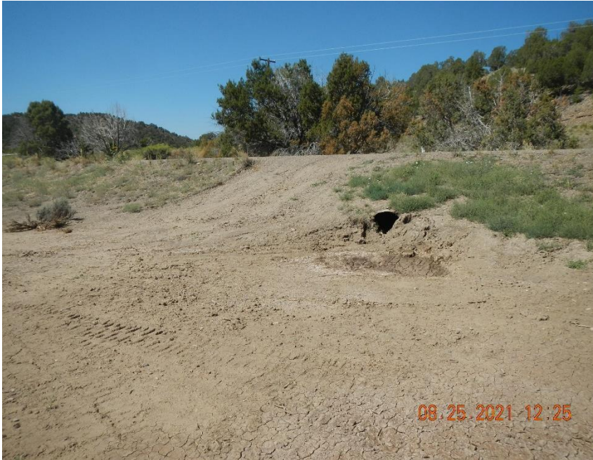
Outlet of culvert beneath dirt road.
