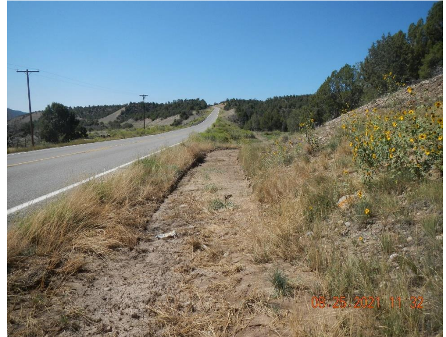
Initial actions included scraping up impacted material from along flow path.
