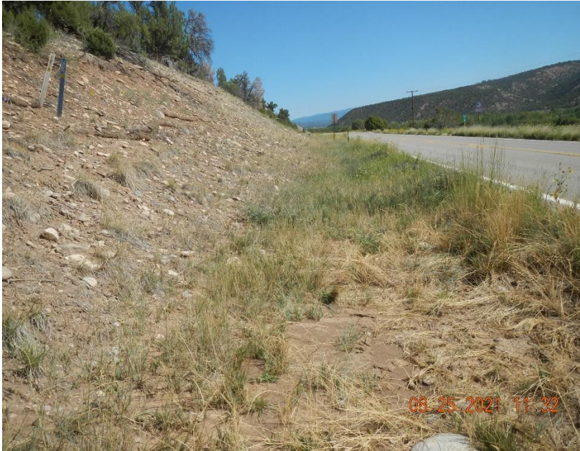
Point source of Spill/Release Point ID #480312 on hillside adjacent to Highway 151.
