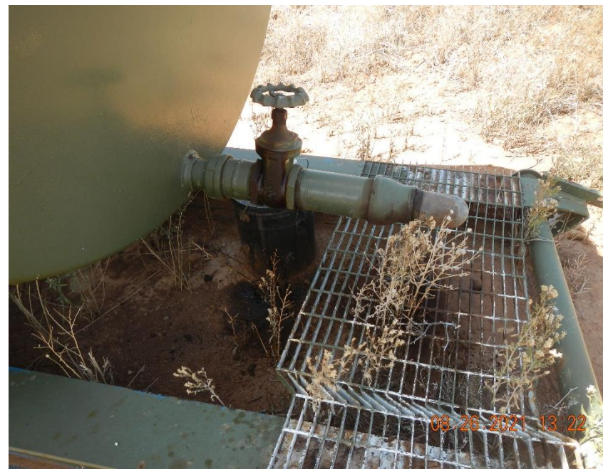
Truck load out valve on horizontal tank is wet and stained with oil. Soil beneath valve is wet and stained.
