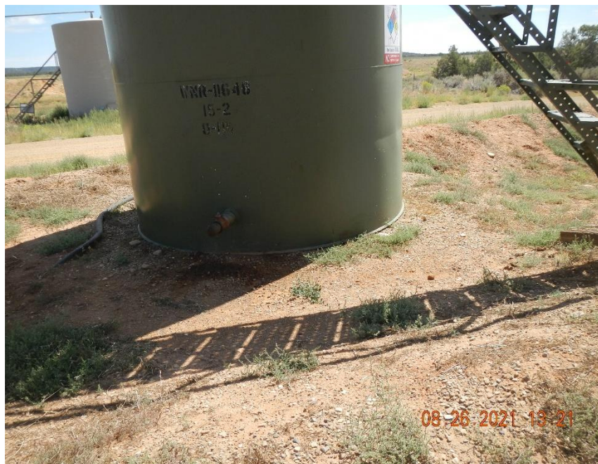
Stained soil beneath truck load out valve.
