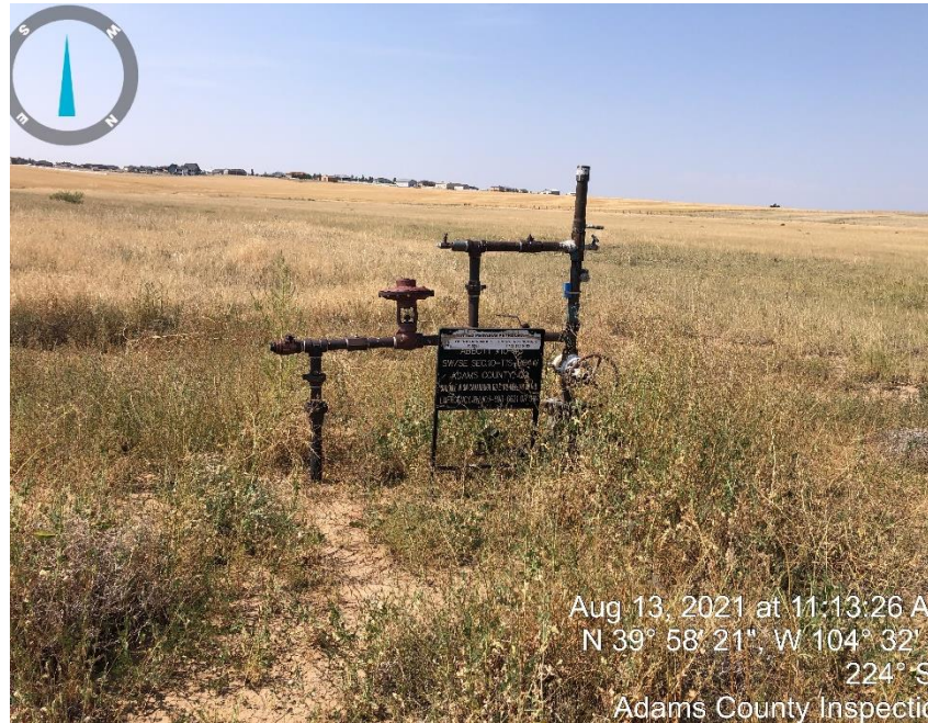
Photo #1 Well Head.
