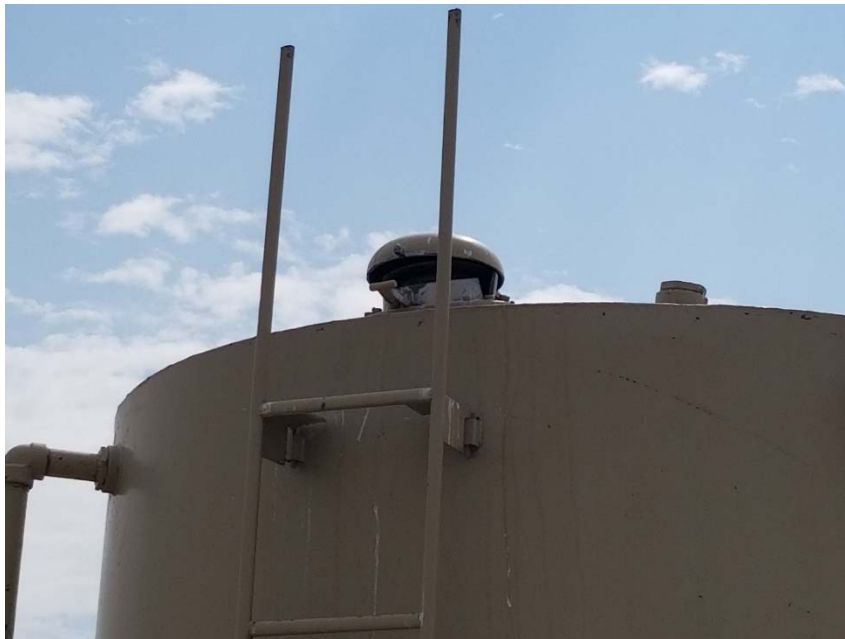
Photo 5. Gauge hatch open.
