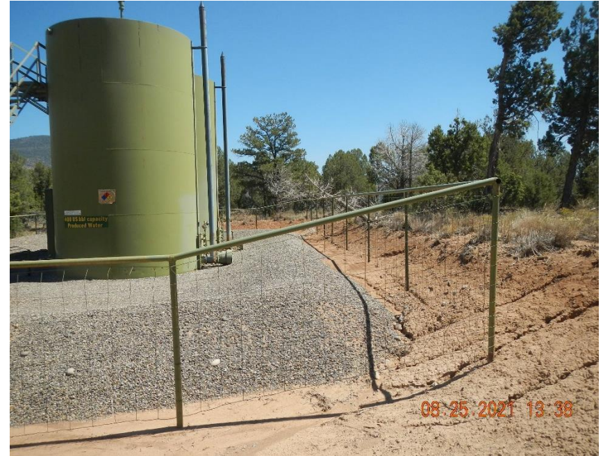
Sediment deposited on location from cut slope on southern edge of location.
