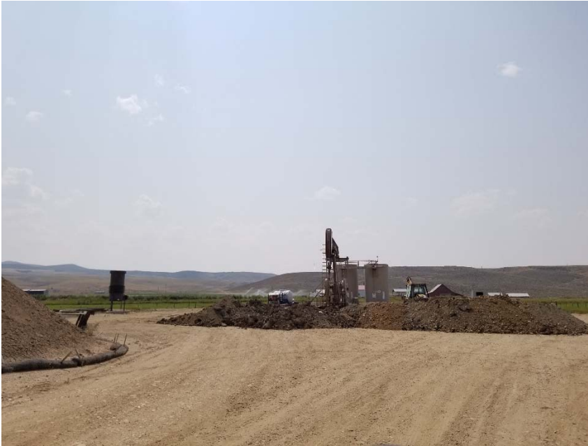
Photo 1. Overview of location taken facing south. No stormwater controls around soil pile from earthwork at wellhead.
