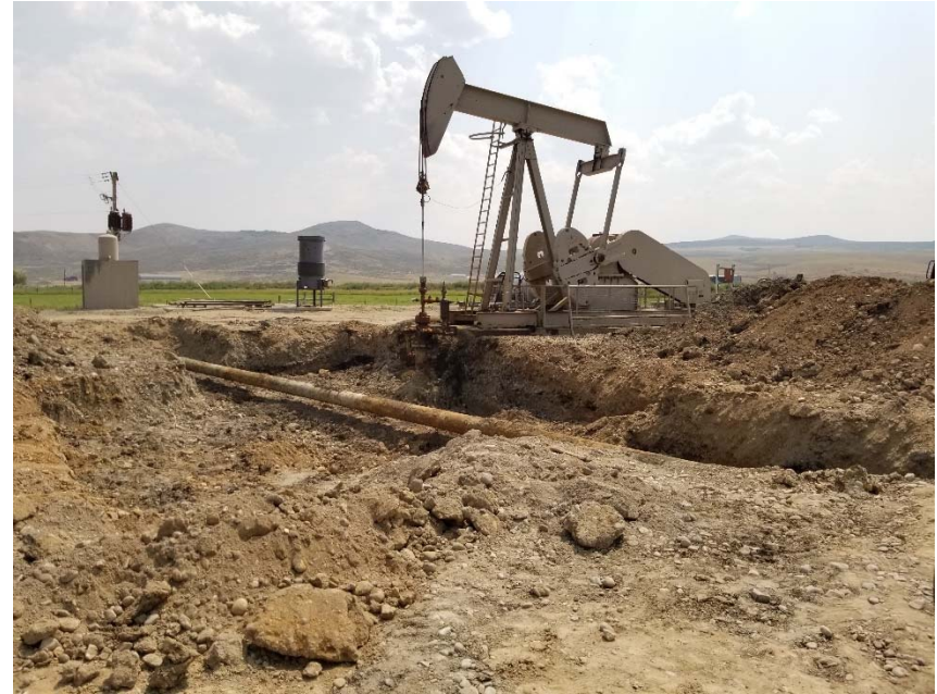
Photo 2. Earthwork at wellhead with no stormwater controls.
