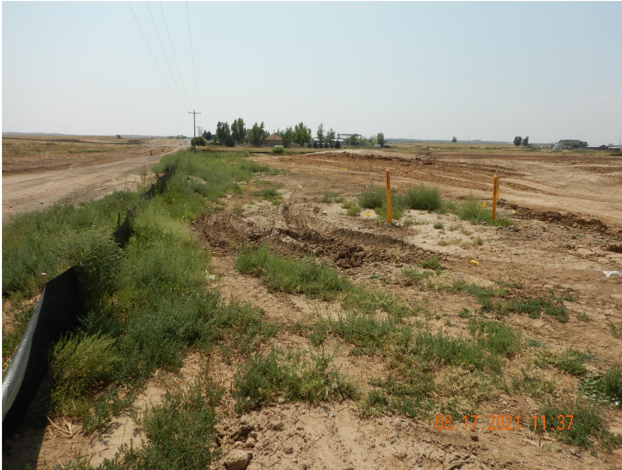
Photo 4. Photo taken from the associated offsite tank battery, facing South. Photo illustrates all equipment has been removed. See comments under Photo 2.
