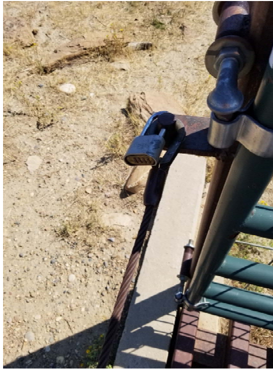
Photo 1. Locked gate at entrance. Please provide gate code to inspector via email.
