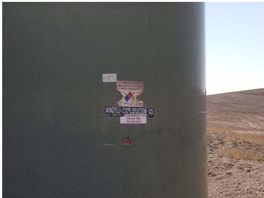
Photo 4. Produced water label peeling.
