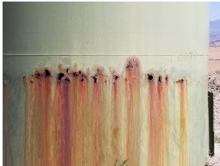
Photo 3. Holes in produced water tank.
