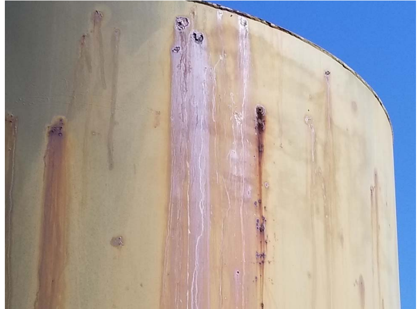
Photo 3. Holes in upper part of produced water tank.
