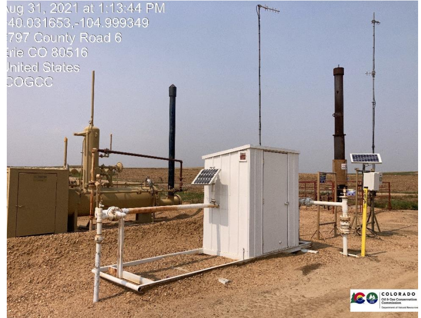
Pic 2 Separator, gas meter run, ECD.
