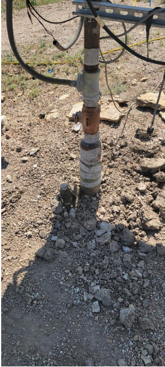
Installed appropriate fittings to allow bradenhead visual inspection as per Rule 419.a.(1), (2).
