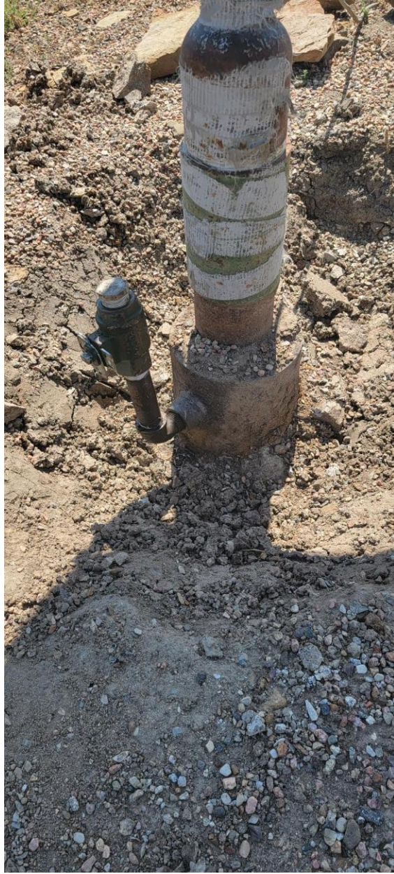
Installed appropriate fittings to allow bradenhead visual inspection as per Rule 419.a.(1), (2).
