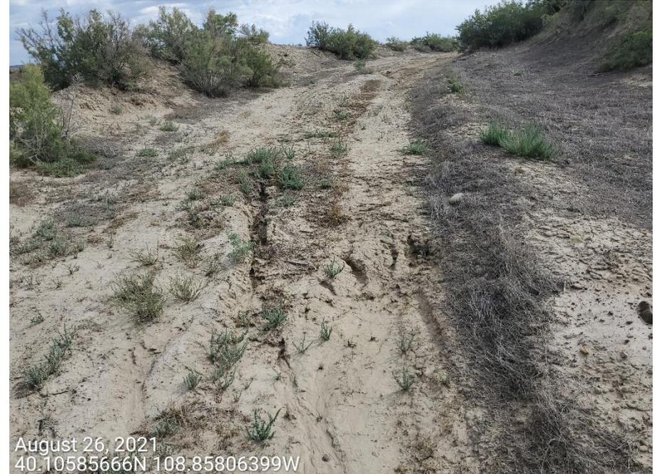
**Photo 4:** Photos taken from the access road. Photos provide example of stormwater erosion observed on the Location.
