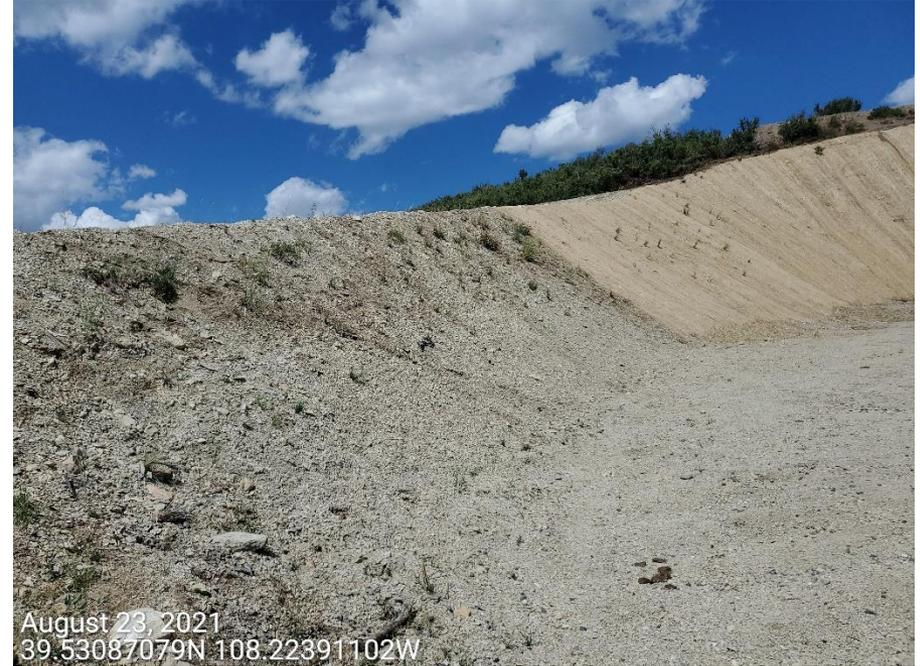
**Photo 2:** Photos provide example of areas on the north and west end of the Location, where BMPs to protect and stabilize the slopes remain missing or insufficient.
