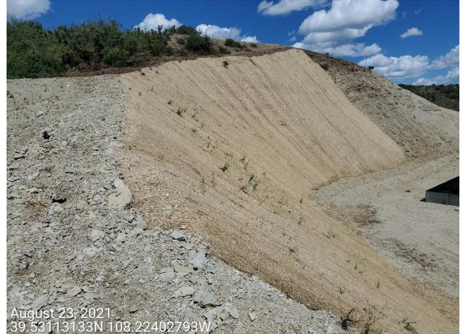
**Photo 1:** Photos provide example of BMPs (erosion control blankets) that have been installed to protect and stabilize the slopes on the north and west end of the Location.
