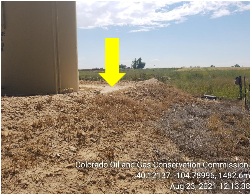
Photo 7 breach in secondary containment berm.
