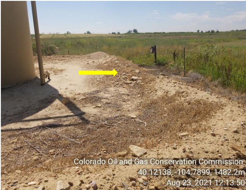
Photo 9 Breach in secondary containment berm.
