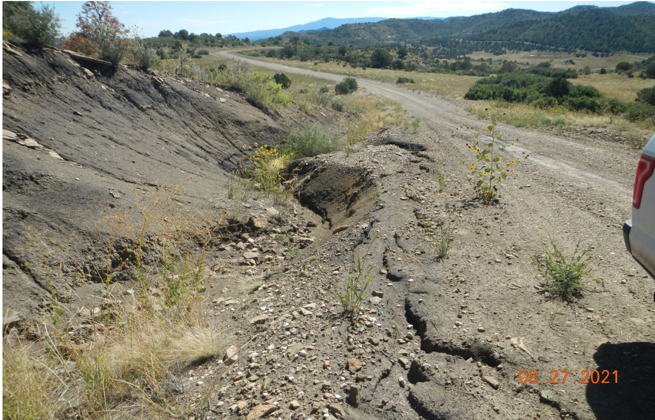
Photo 1. Facing east along the main road traveling to the well site. There is erosion along the road side. This area needs to be repaired and stabilized.
