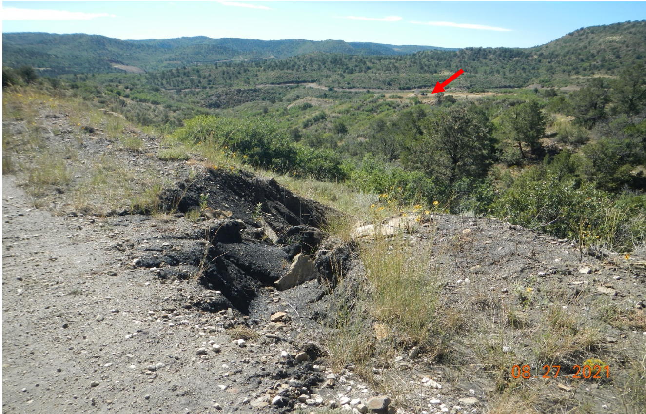
Photo 2. Facing southeast along the main road traveling to the well site. There is erosion along the road side. This area needs to be repaired and stabilized. Red arrow points to the well site.
