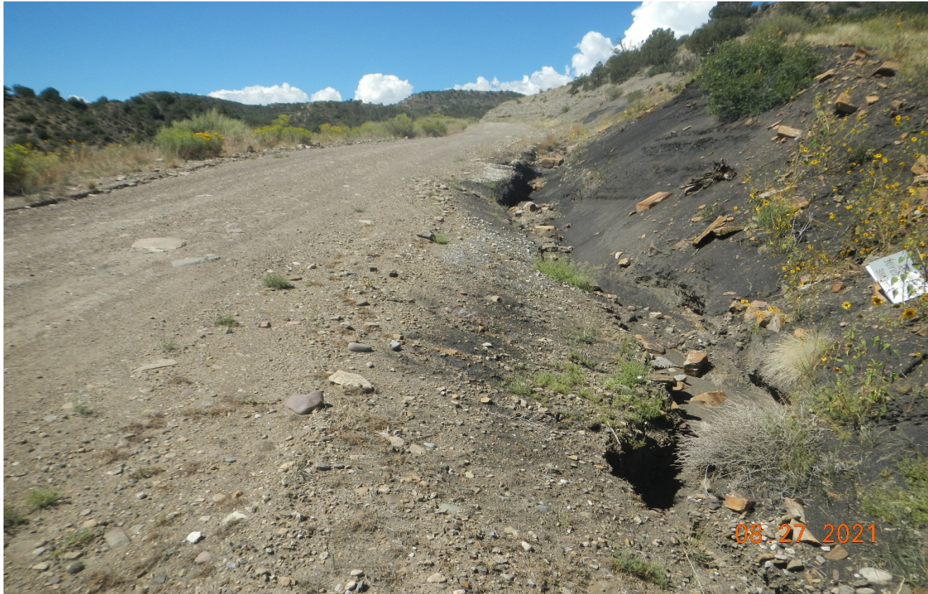
Photo 1. Facing southwest along the main road to the well site. There is erosion along the road which is causing sediment accumulation at the culvert and at the main road in Lorencito Canyon.
