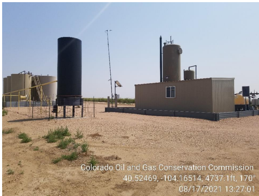
Photo 3 – Heater Treater and ECD
