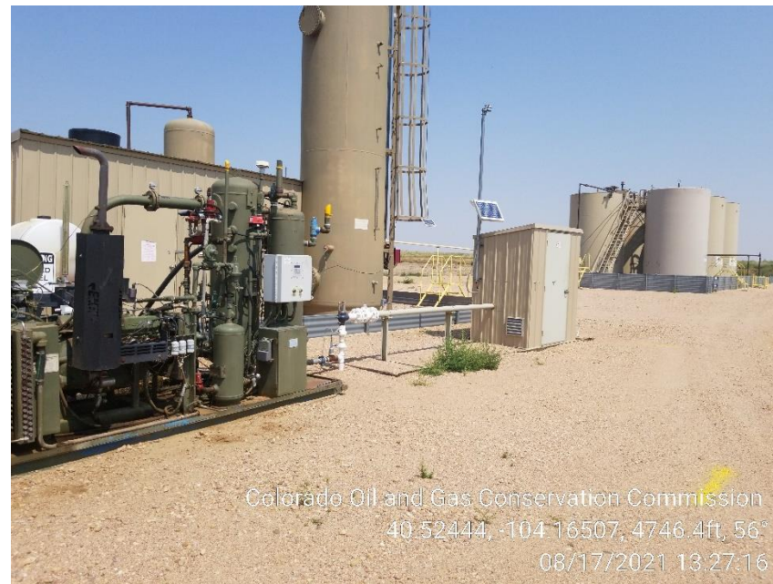
Photo 4 – Sales Compressor and Gas Meter
