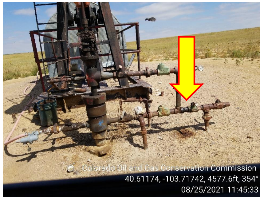
Photo 2 – Wellhead – Stained Soil/Leaking Valve
