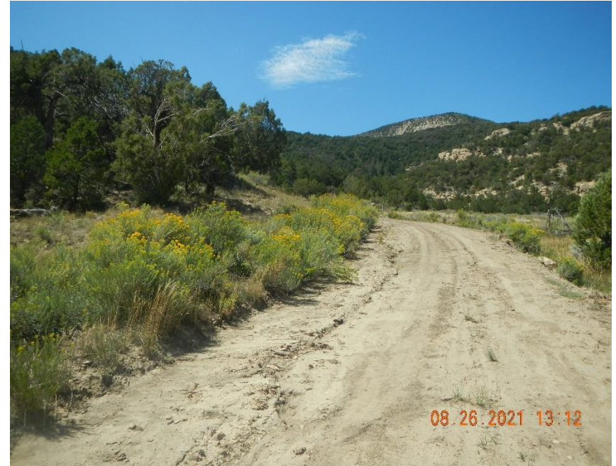
Storm water rill on access road.
