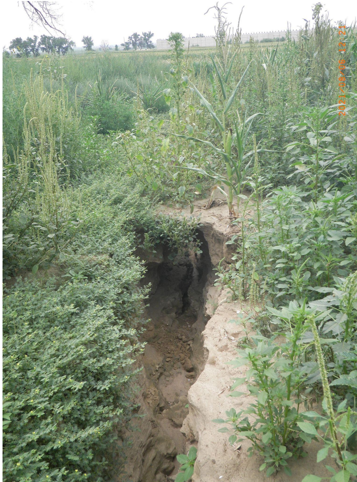
Photo 4. Photo along western edge of tank battery (looking southwest). Photo illustrates channelized flows that are causing gully erosion adjacent to the site. See comments in photo 3.
