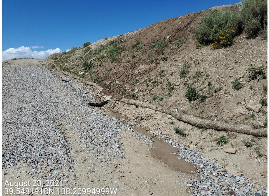
**Photo 3:** Photo taken south end of the Location. Photo shows BMPs to protect and stabilize slopes of the Location, and to allow for sediment laden-free stormwater discharge, remains missing or insufficient.
