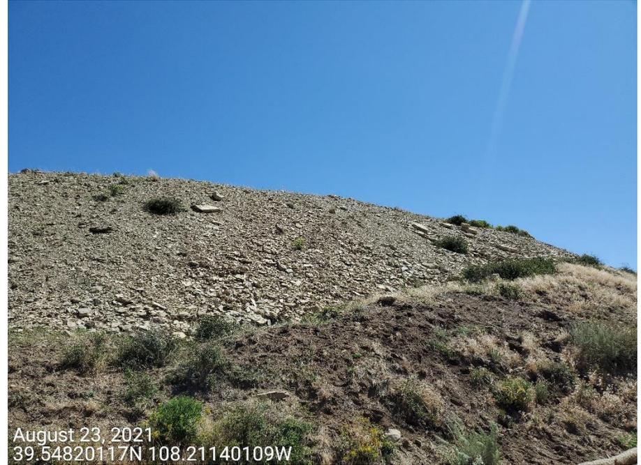
**Photo 5:** Photos show examples of the cut/fill slopes on the Location, where BMPs to protect and stabilize the slopes are missing or insufficient
