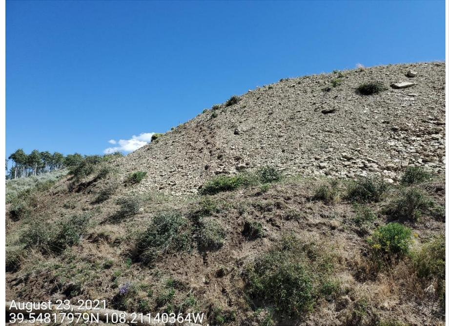
**Photo 4:** Photos show examples of the cut/fill slopes on the Location, where BMPs to protect and stabilize the slopes are missing or insufficient.
