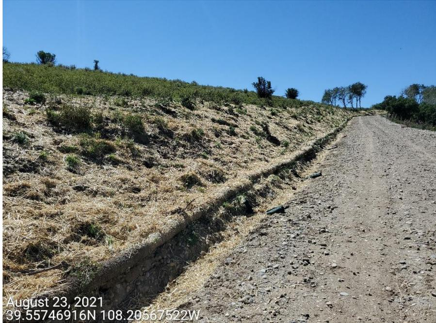
**Photo 3:** Photo taken from the access road. Photo shows additional control measures to stabilize and protect slopes along the access road have been installed.
