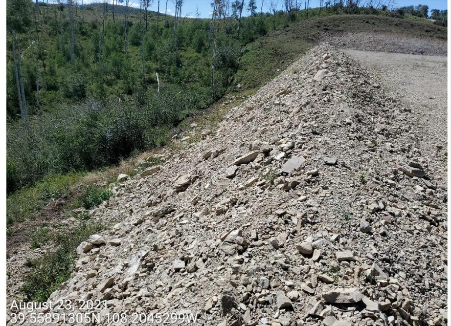
**Photo 2:** Photos taken from the slopes on the east and west end of the Location. Photo shows control measures to protect and stabilize the slopes of the Location remain missing or insufficient.
