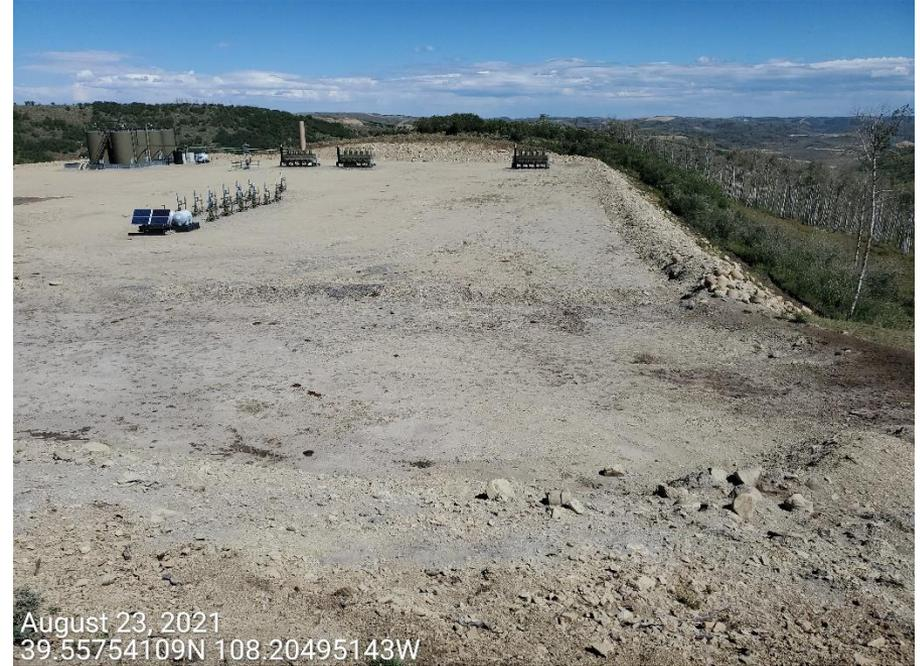
**Photo 1:** Photos taken from the southeast end of the Location. Photos provide overview of the Location. Photos show interim reclamation of the Location has not been conducted in accordance with 1003 Rules.
