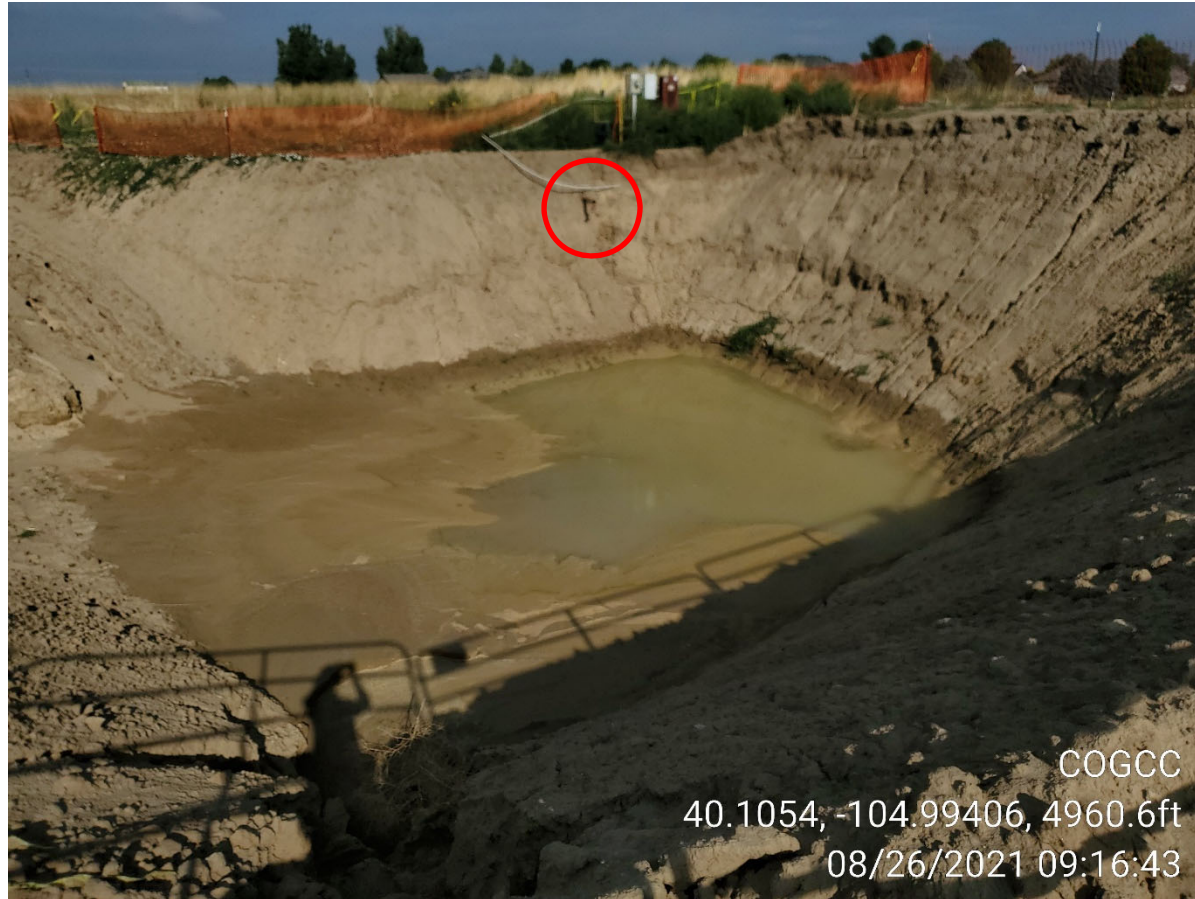
Photo 2: Excavation from southeast corner, looking northwest. Flowline exposed in northwest corner of excavation – highlighted by red circle.
