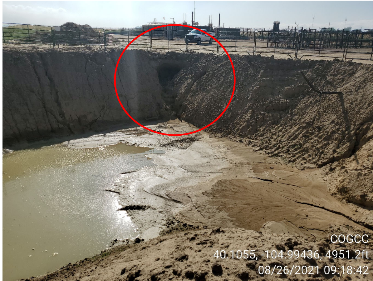
Photo 9: Northwest corner of excavation looking along southeast. Erosion of southeast corner visible.
