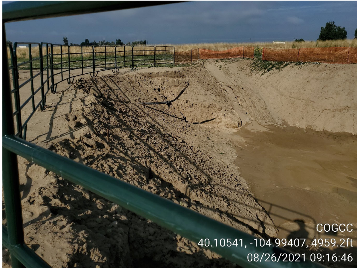
Photo 3: Excavation from southeast corner, looking west. Flowline exposed in south wall of excavation.
