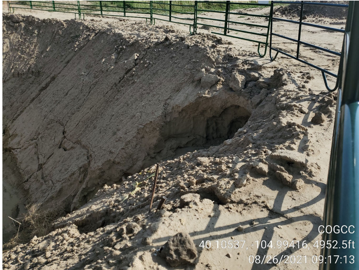
Photo 5: Excavation looking at southeast corner. Erosion of excavation wall in southeast corner.
