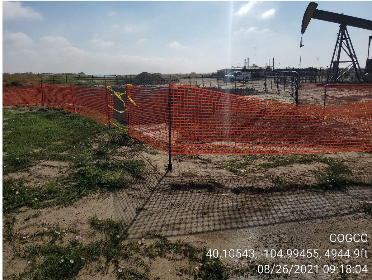
Photo 7: Excavation from northwest corner looking east. Fencing is a combination of cattle panels, snow fence and caution tape.
