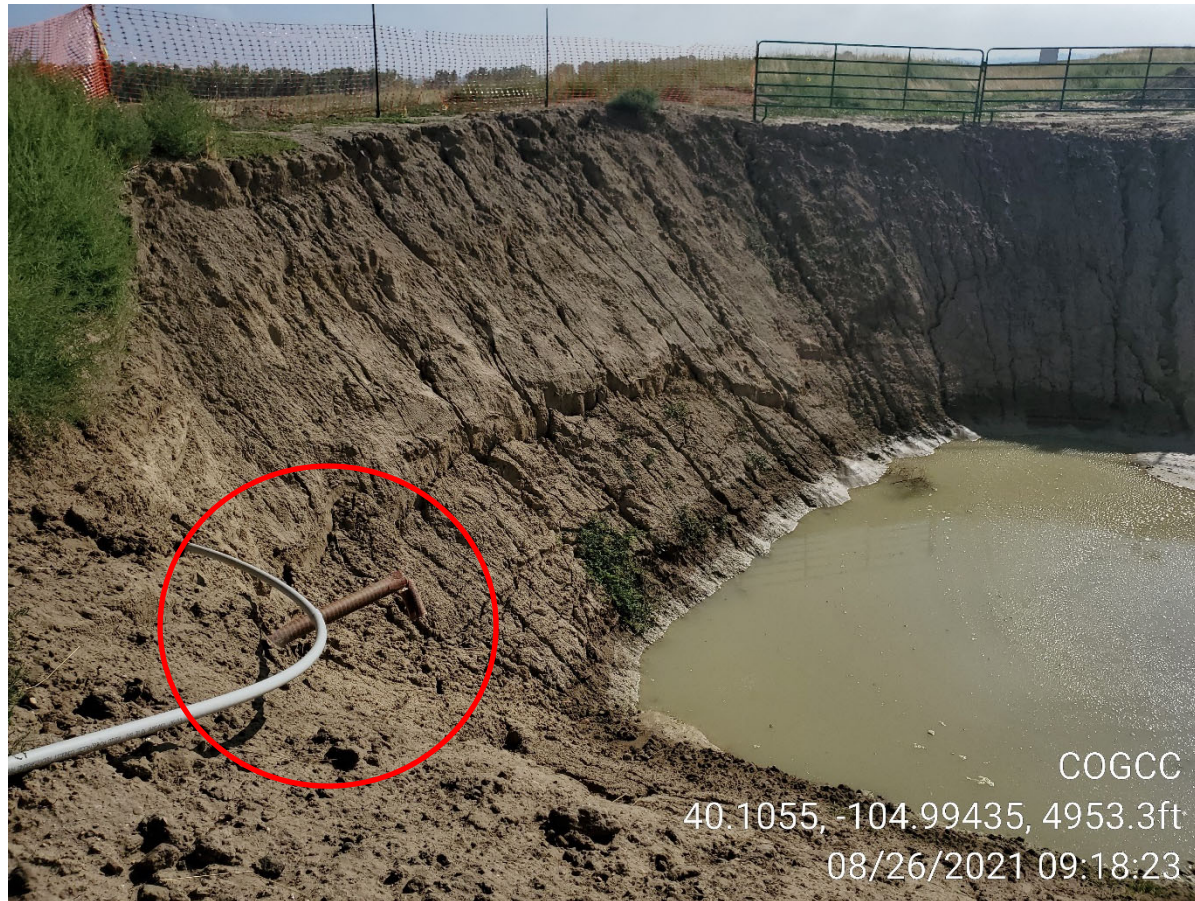
Photo 8: Northwest corner of excavation looking along north wall. Flowline is exposed in northwest corner of excavation (highlighted by red circle).
