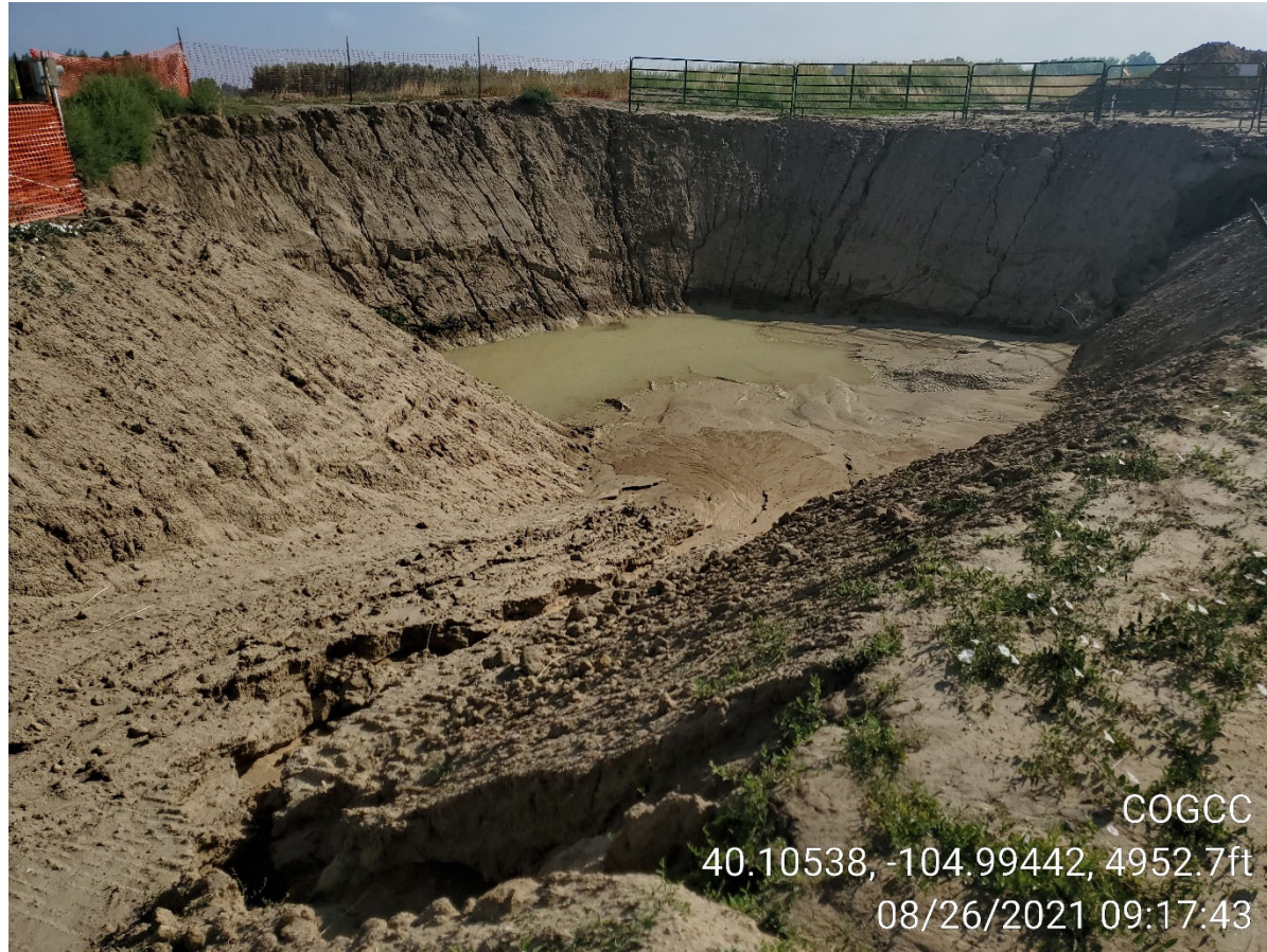
Photo 6: Excavation from southwest corner. Erosion is occurring in foreground, and in southeast corner in upper right of photo.
