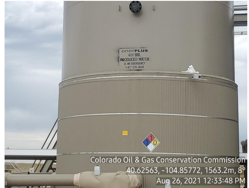
Photo 4: NFPA placard installed
