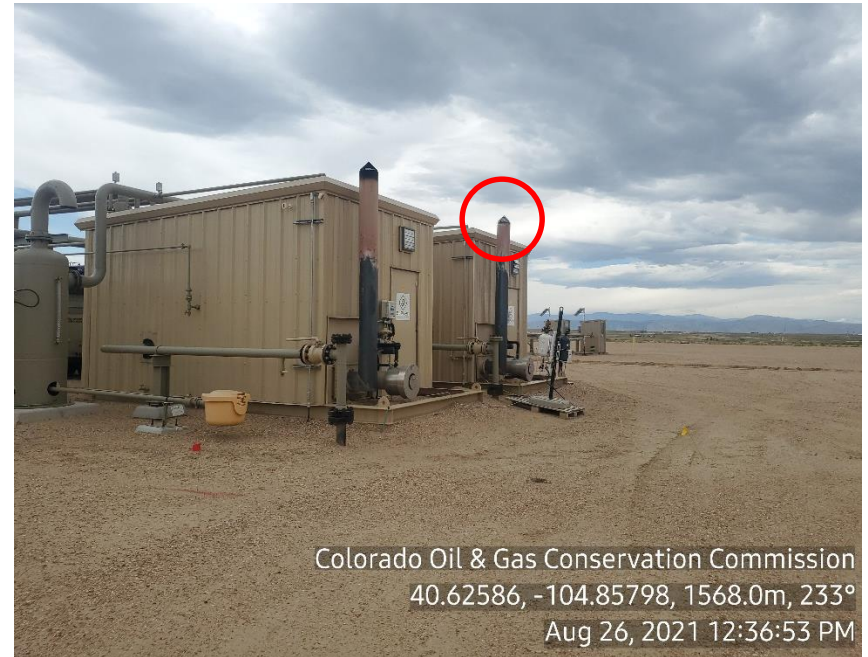
Photo 2: Bird protector installed
