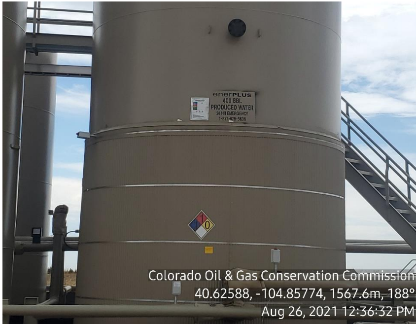
Photo 3: NFPA placard installed
