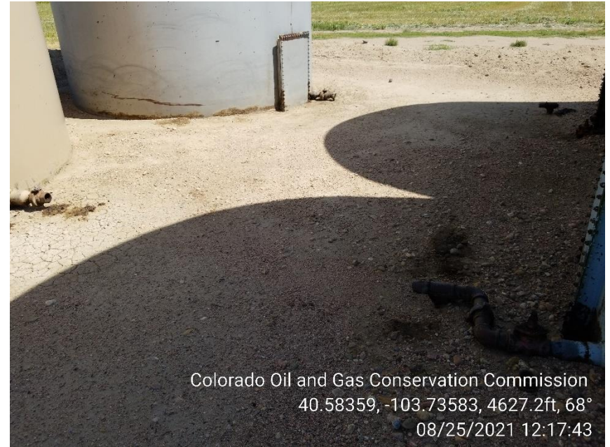
Photo 8 – Stained Soil at Drain Valves
