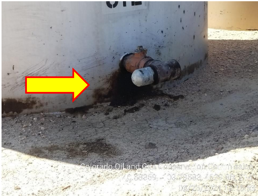
Photo 7 – Stained Soil at NE Loadline
