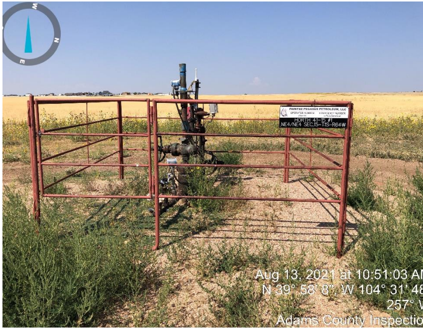
Photo #3 Well Head.
