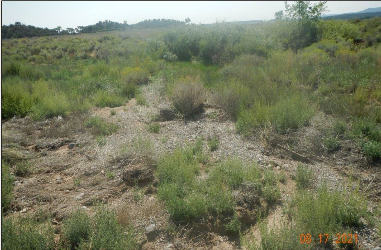
Photo 5. View of gravel and sediment discharged from overflow of stormwater downstream from the access road (area approx. 15ft wide x 25ft long)
