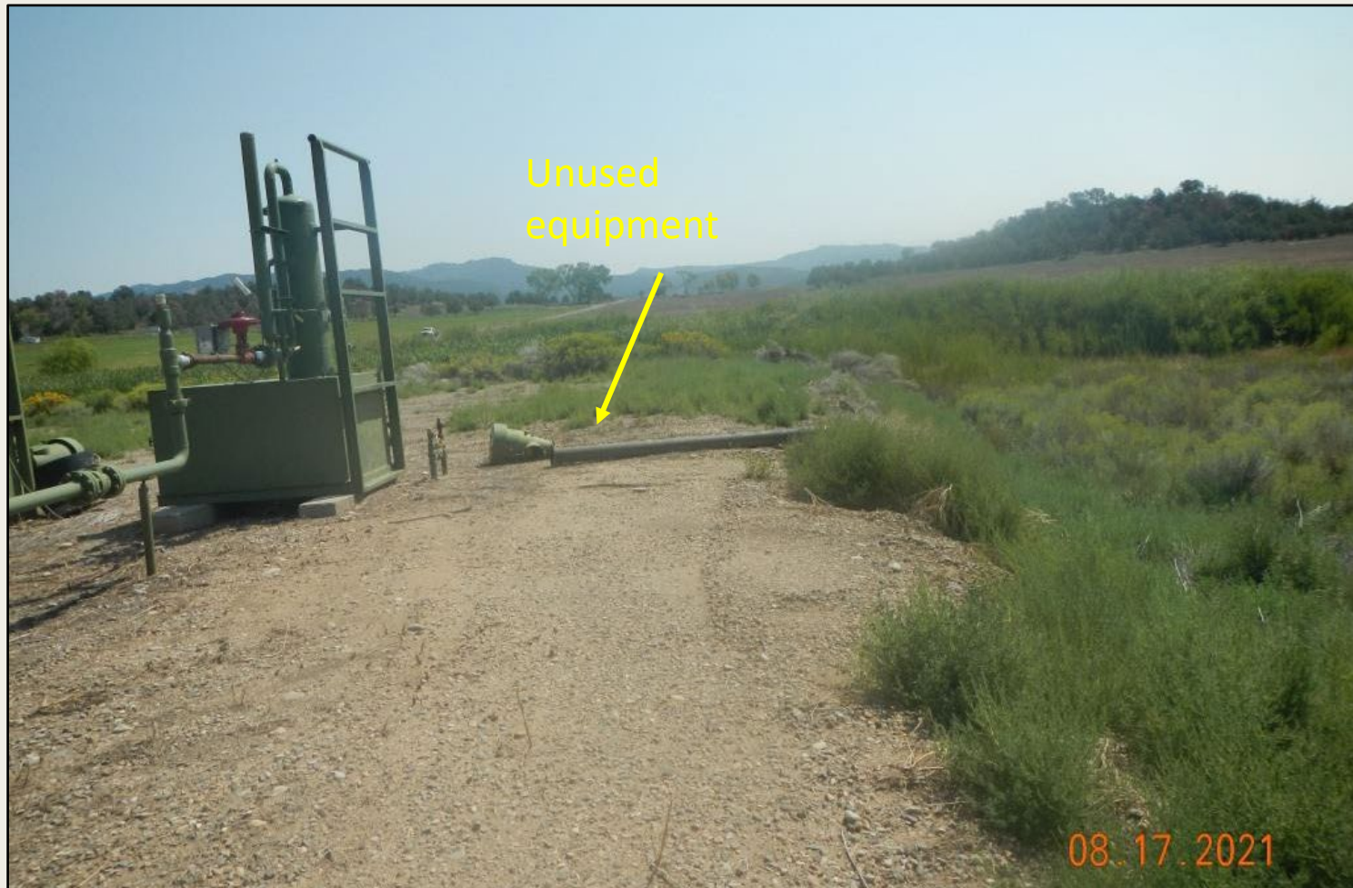
Photo 3. View of the southern project area facing eastward. Revgetation is progressing on fill slopes, largely with rubber rabbitbrush. Kochia weeds need to be managed to prevent debris. Unused equipment also present here.
