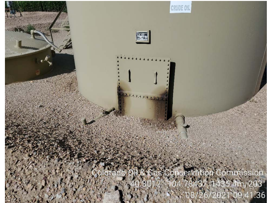
Clean out plate and stained soil
