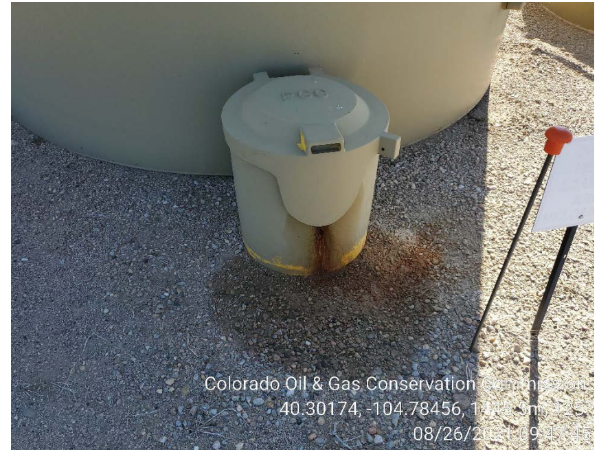
Load valve drip bucket and stained soil
