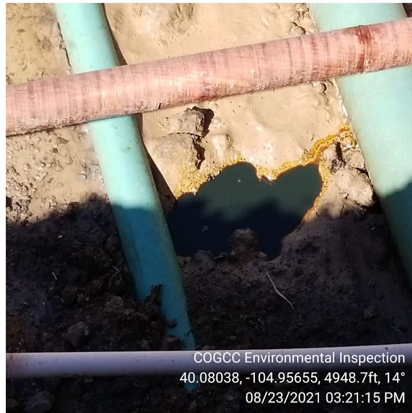
Photo 2 – Excavation floor. Free product visible on water.
