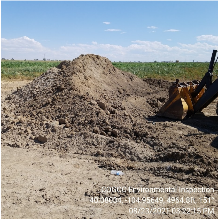
Photo 5 – Impacted soils stockpiled. Inadequate stormwater controls.
