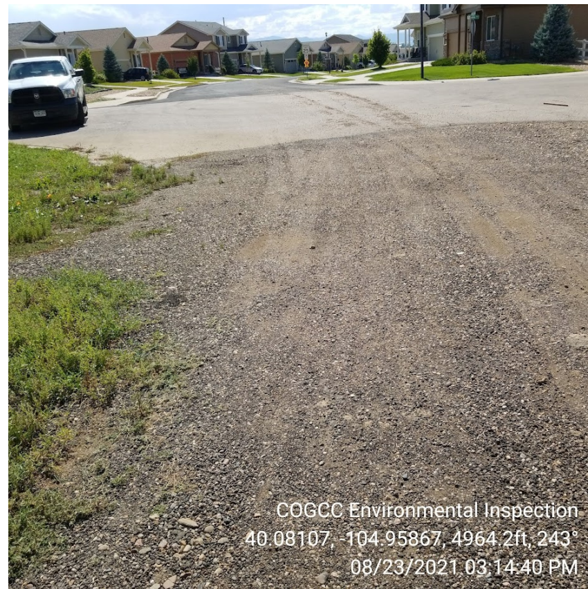
Photo 8 – Vehicle tracking onto residential roads.
