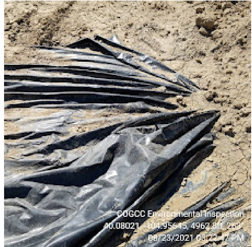
Photo 6 – Liner under stockpiled soil is damaged.
