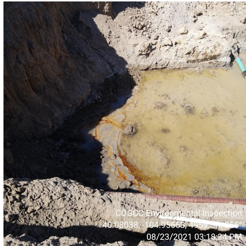
Photo 4 – Floor. Free product visible on water.
