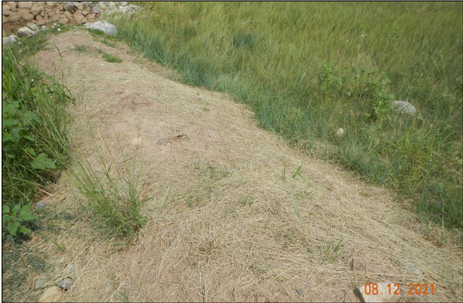
Photo 4. View of hay mulch on berm and germination observed.
