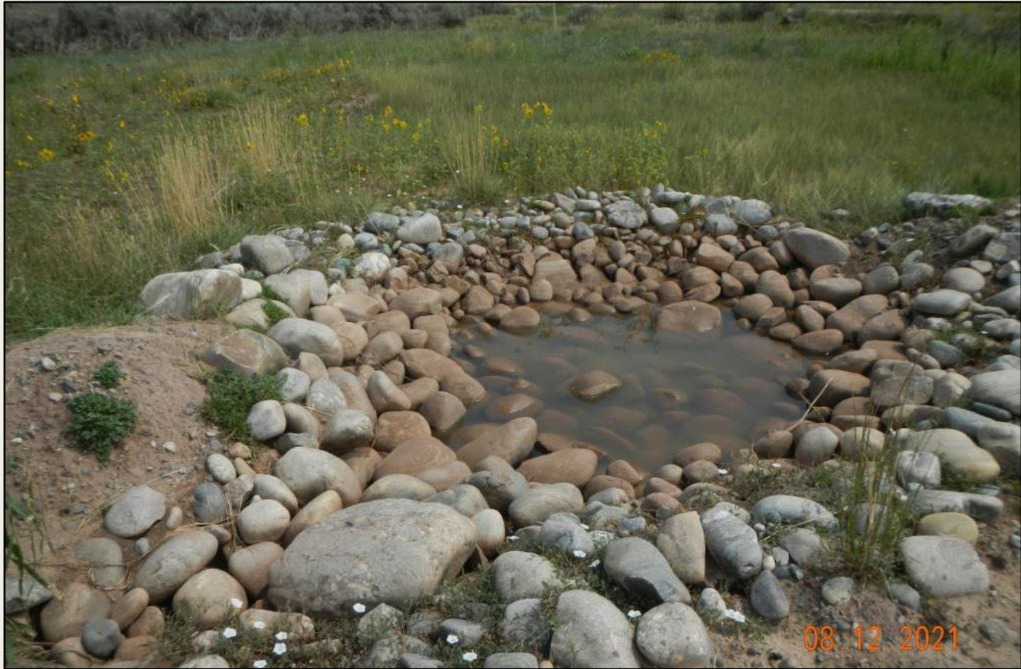
Photo 3. View of silt trap observed within the northern project area.
