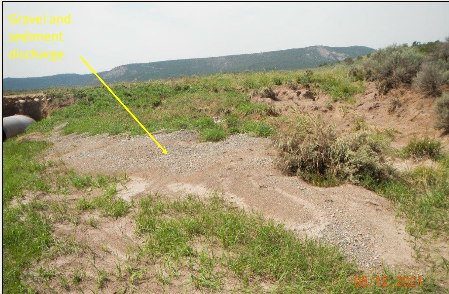
Photo 4. View of gravel, road, material and scoured soils downstream from area where stormwater event flowed over the access road. Sediment discharge in this area is approximately 25 feet long and 4 feet wide, depth unknown.
