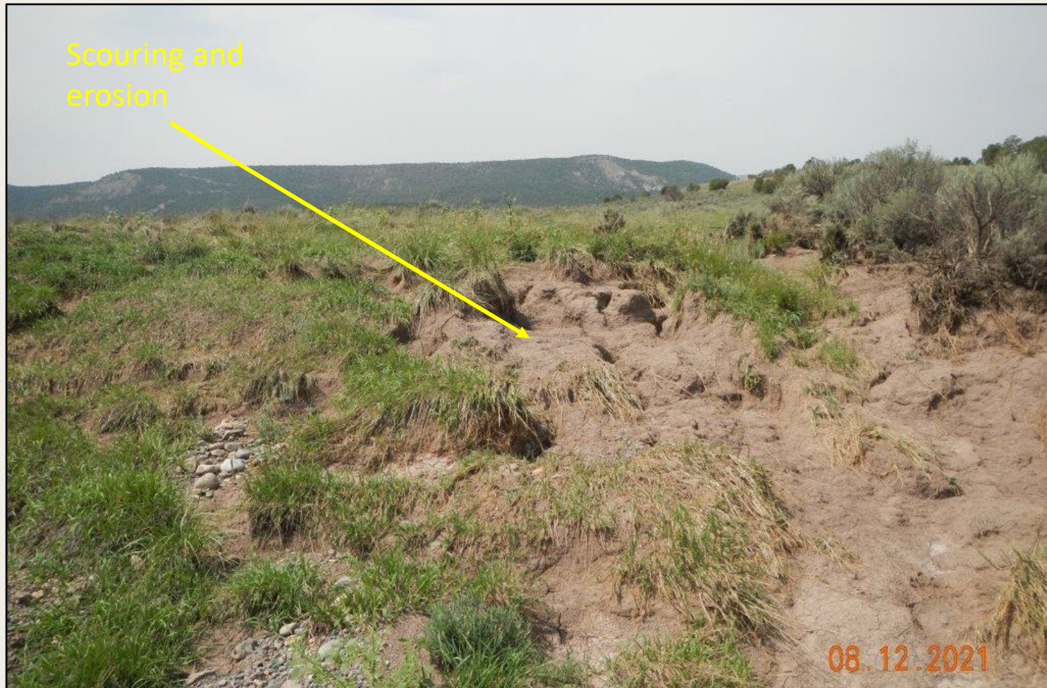
Photo 5. View of scouring and erosion on soils down-slope from the access road.
