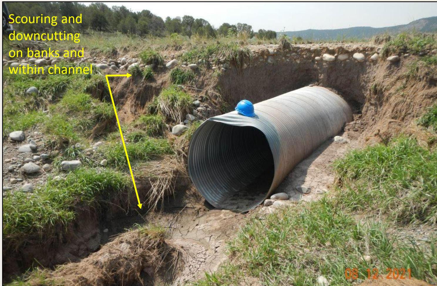
Photo 3. View of erosion occurring at culvert outlet along access road, indicating that this culvert is not adequate to support flows in this drainage. An area approximately 3ft x 8ft volume of material is eroded around the culvert, as well as scouring and transport of road materials.
