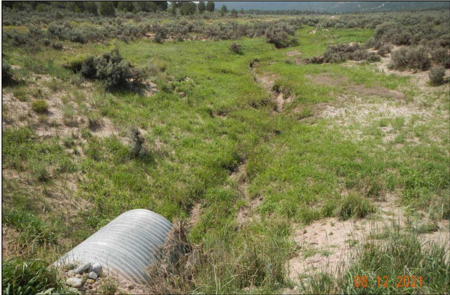
Photo 6. View of culvert inlet on upstream side of access crossing. Significant erosion is not observed upstream from access road crossing.
