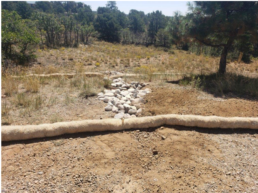
Installed erosion stabilization.
